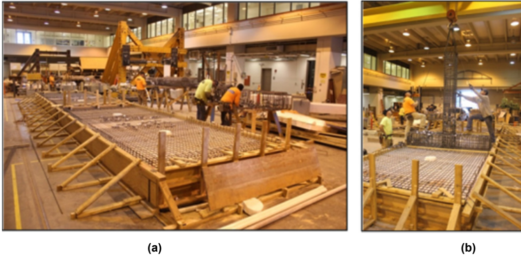
Figure 3.17 (a) Reinforcement steel mesh for the deck slab and (b) fabrication and setting up of the column and cap beam steel cages.
