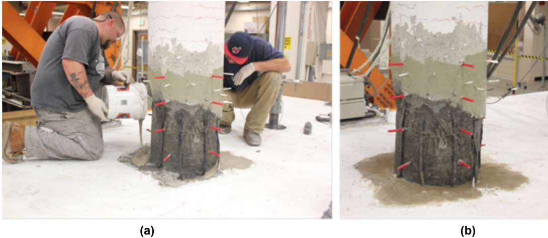
Figure 6.6 (a) Partially fixing the column-bent cap interface using a sand-epoxy mixture; and (b) overview of the partial repaired column after installing all injection ports, CFRP reinforcing bars, and patching the damaged parts in column core and at the column-bent cap interface.
