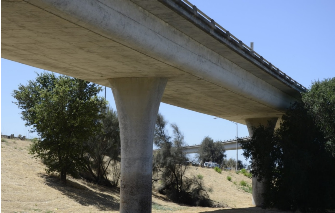
Figure 1.2 Typical California box-girder bridge: W80-E50 Connector Overcrossing, Yolo County, California (photo courtesy of Mark Yashinsky, Caltrans).
