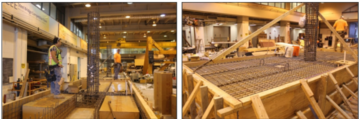
Figure 3.19 (a) Installing custom-made cardboard boxes for box-section and (b) furnishing reinforcement steel mesh for the soffit slab.
