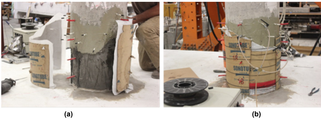
Figure 6.7 (a) Installing the sonotube around the damaged zone to restore the column's circular shape; and (b) injecting fluid epoxy into the cracks using the installed injection ports.
