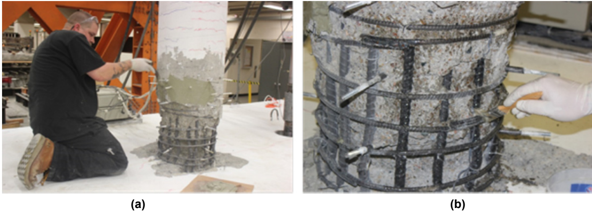
Figure 6.3 (a) Installing the injection ports along the cracks and patching the concrete surface around the ports; and (b) exposed rebars coated with epoxy primer for better bond.
