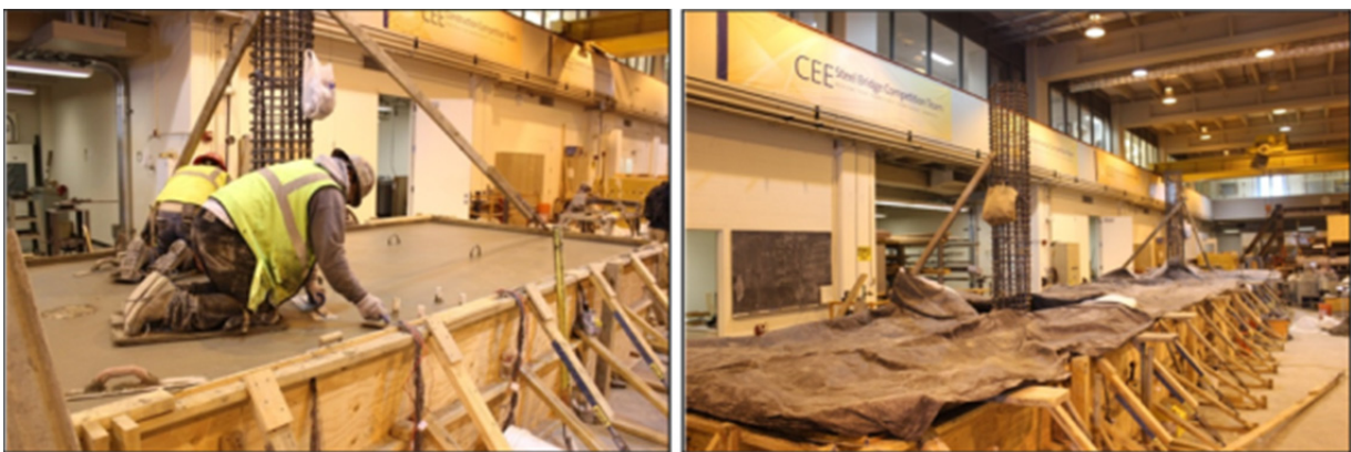
Figure 3.19 (a) Installing custom-made cardboard boxes for box-section and (b) furnishing reinforcement steel mesh for the soffit slab.
