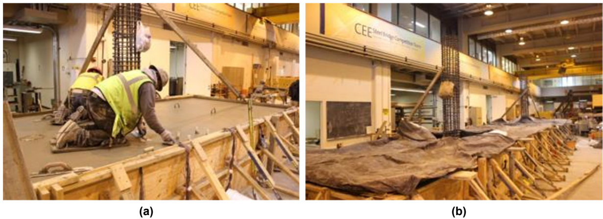
Figure C.10 (a) Finishing the surface of the second concrete lift; and (b) using curing blankets in addition to the E-CURE to avoid any shrinkage cracks in the soffit slab.
