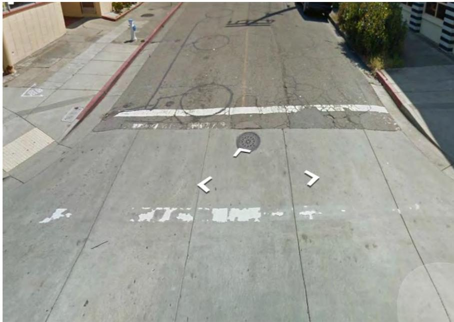
**Figure 33. Example of “Faded” Crosswalk Condition**
