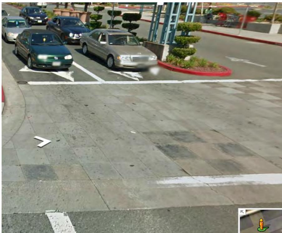
**Figure 32. Example of “Partially Worn” Crosswalk Condition**
