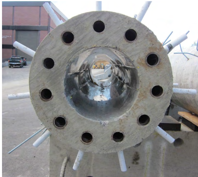
Figure 3.18- GCDP Precast Hollow Column w/ Embedded Sleeves
