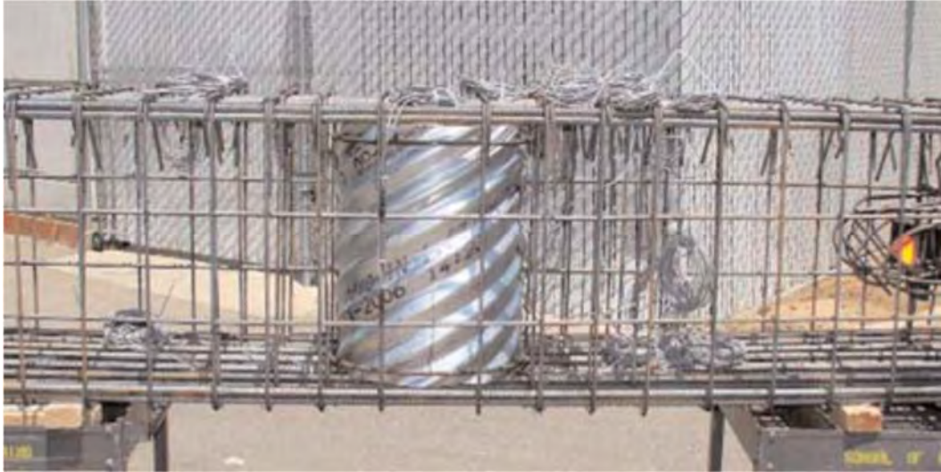
(a) Corrugated Duct Placed in Cap Beam (Elevation)
