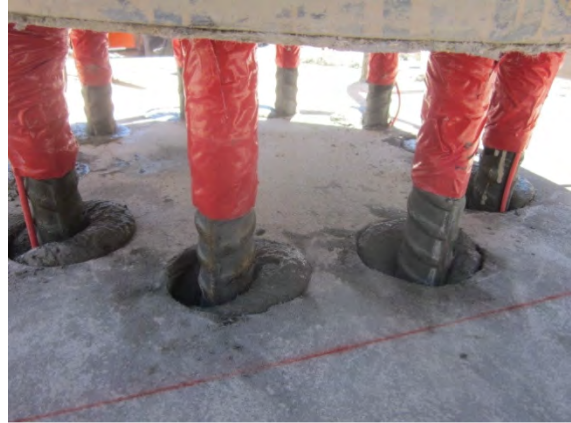
Figure 3.31- HCS Column Shell Installation
