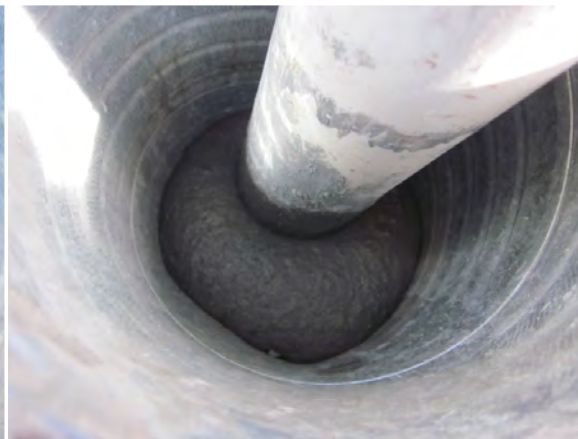
(b) Inside View of Duct During Casting UHPC
