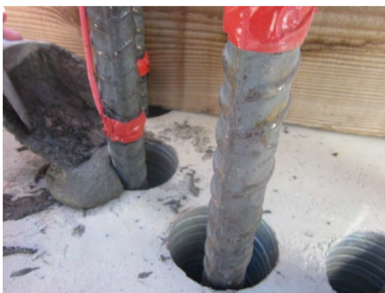
Figure 3.30- Filling Ducts w/ UHPC in HCS Column
