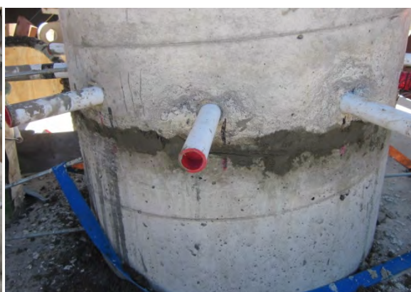
Figure 3.21- Filling Construction Gap w/ Dry Packing
