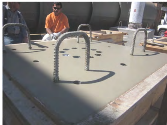
(b) Footing after Casting Concrete
