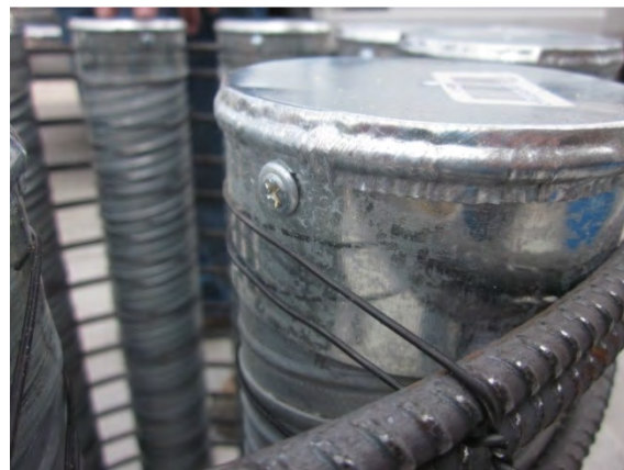
Figure 3.32- Duct Cap for Plugging Duct End
