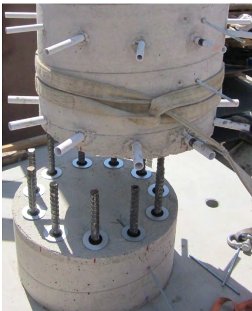
Figure 3.19- Erecting and Installing GCDP Column
