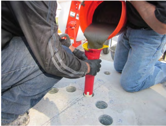
(a) Casting UHPC
