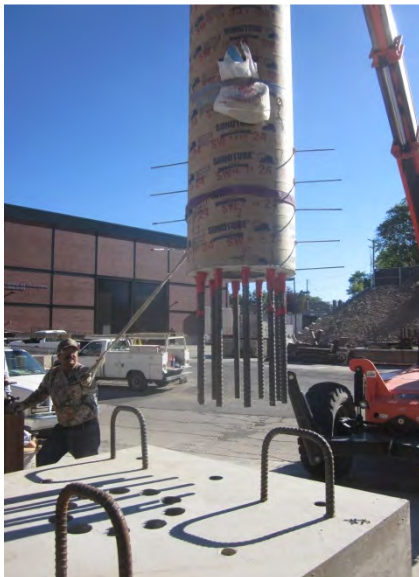
Figure 3.29- Erecting and Securing HCS Column
