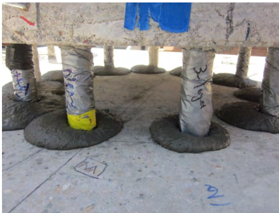
(a) Inserting Reinforcements into Ducts
