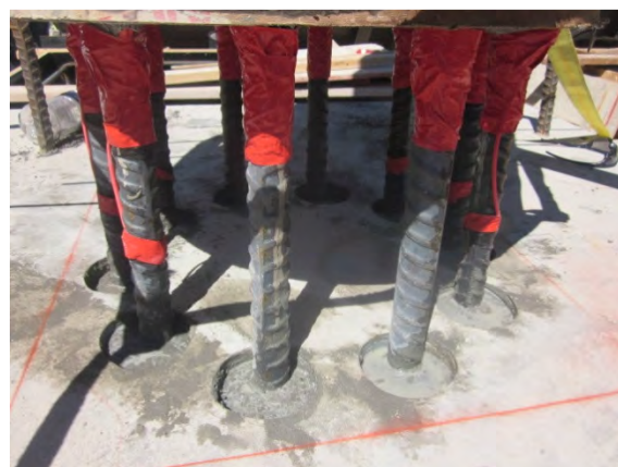
Figure 3.30- Filling Ducts w/ UHPC in HCS Column
