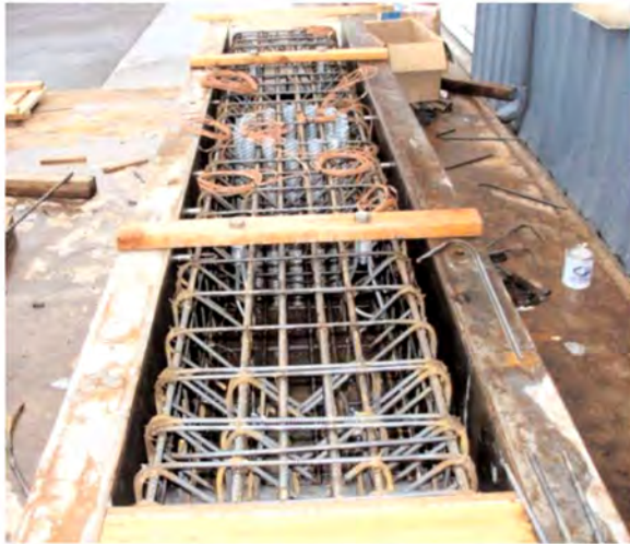
(a) Ducts in Bent Cap Before Casting Concrete
