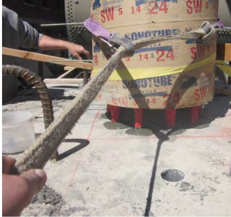
Figure 3.31- HCS Column Shell Installation
