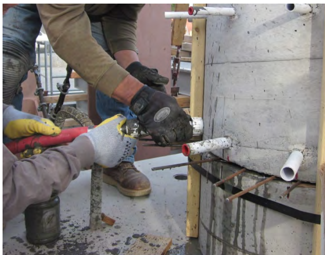
Figure 3.20- Injecting SS-Mortar into Sleeves in GCDP Column
