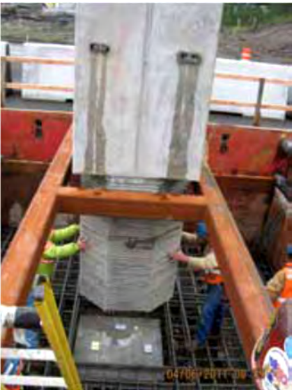
(a) Column Embedded in Footing
