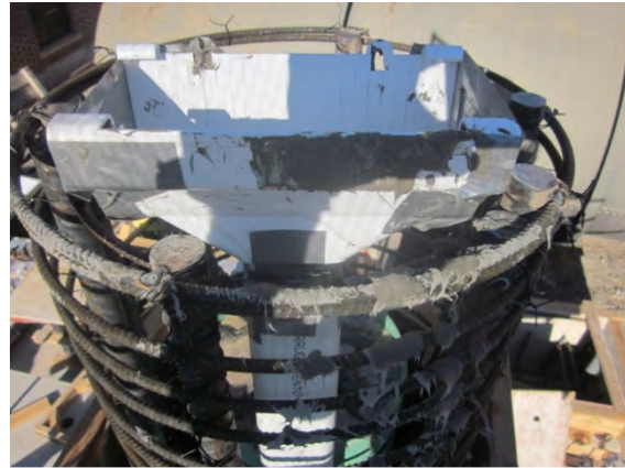
(a) Plastic Gutter Placed at Column Top
