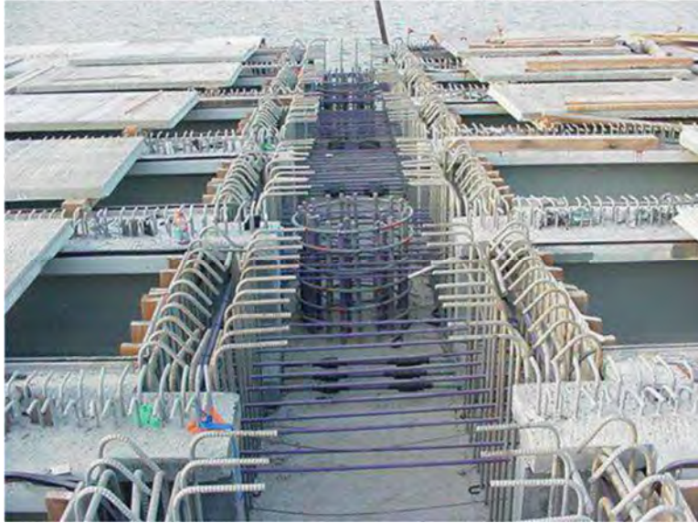
Figure 1.11- Integral Connection (Marsh et al., 2011)
