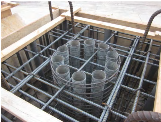
(a) Duct Cage before Casting Concrete
