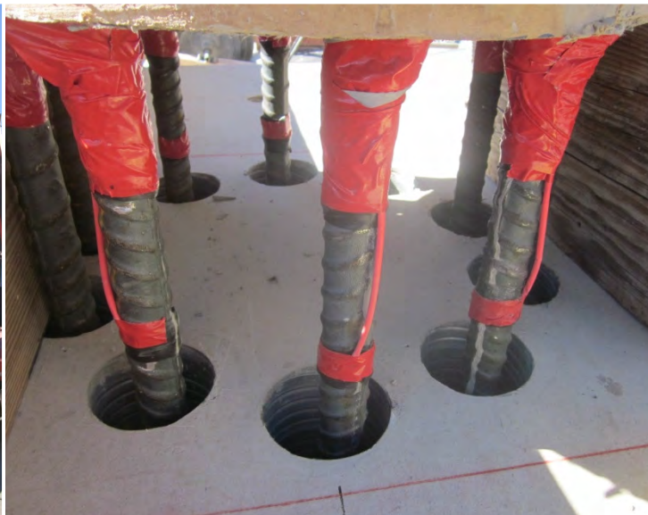
Figure 3.29- Erecting and Securing HCS Column
