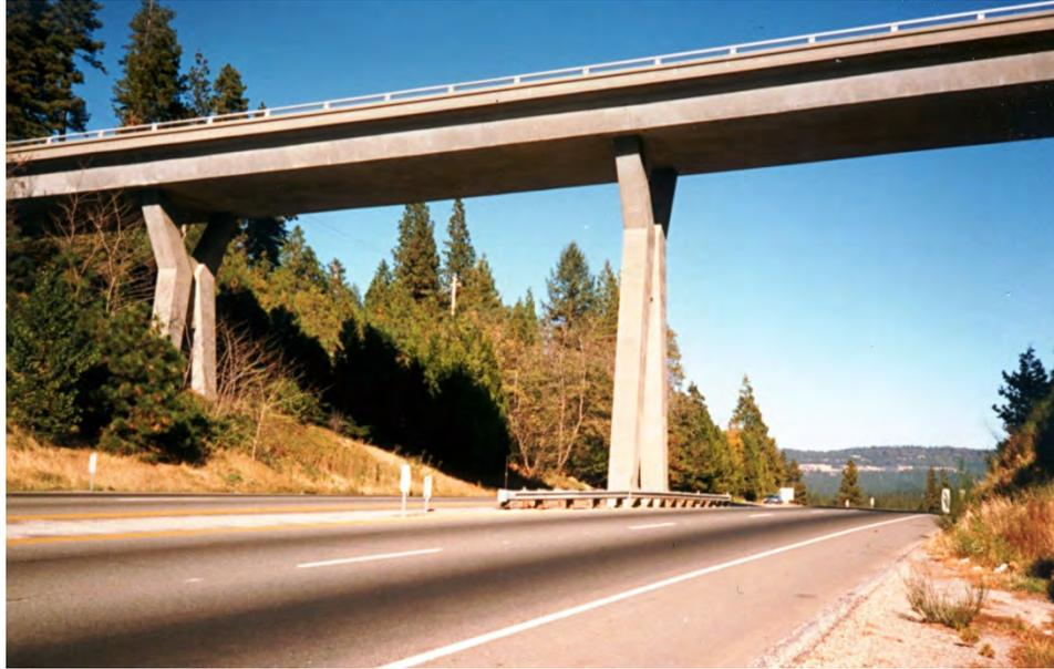
**Figure 1: Concrete box girder bridge in Nevada County, CA (photo by Mark Yashinsky<sup>1</sup>)**
