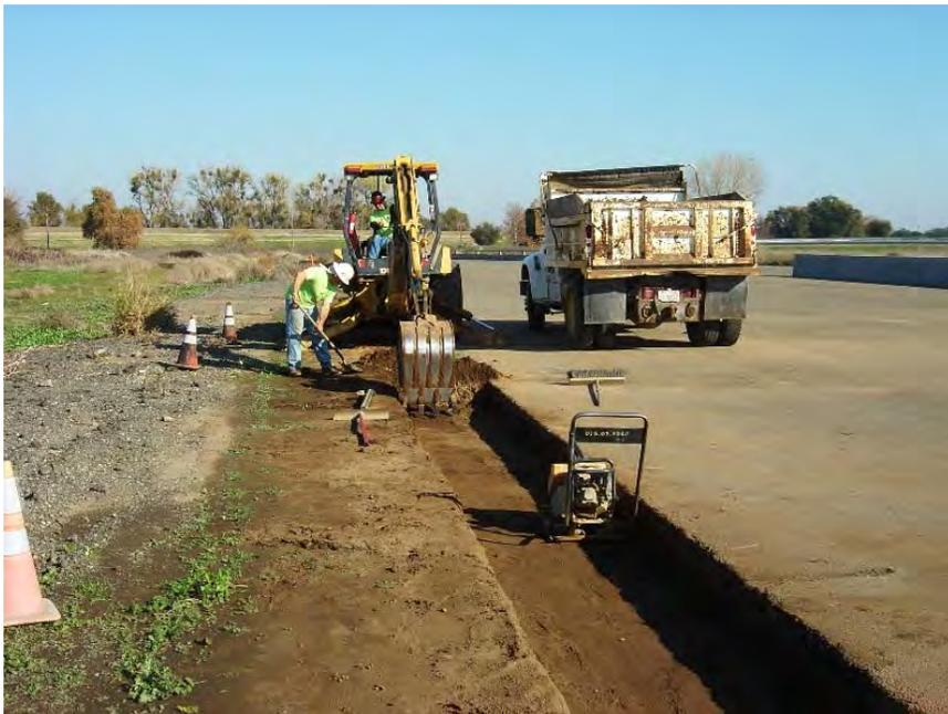
**Figure 2-5. Excavation for Barrier Installation**
