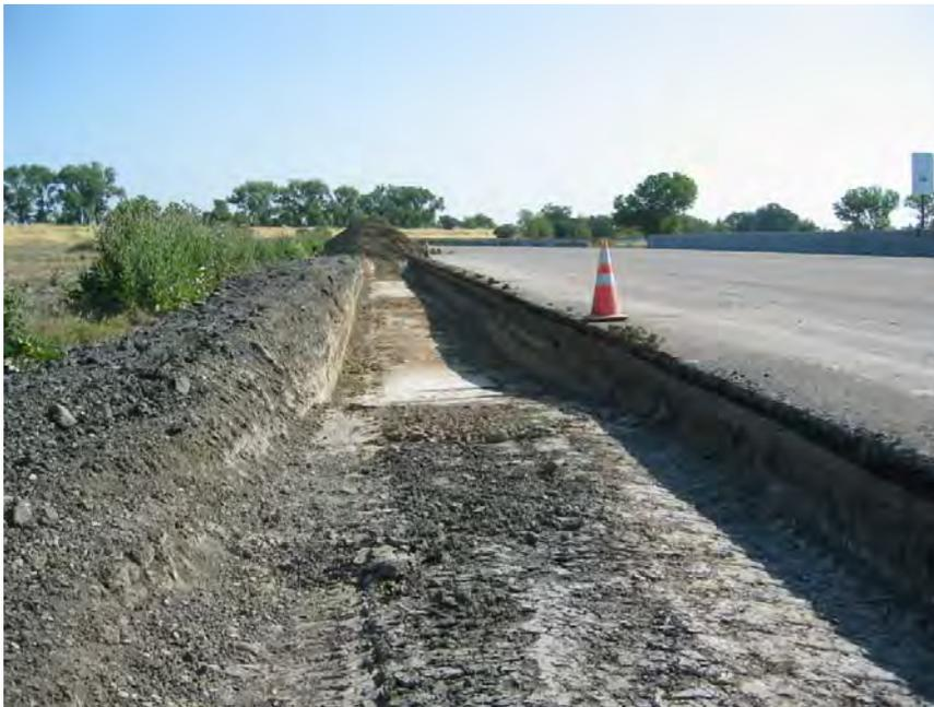
Figure 2-2. Excavation of Existing Soil
