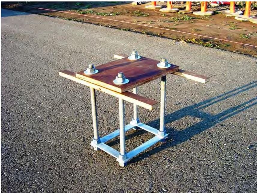
**Figure 2-7. Post Anchor Setup**
