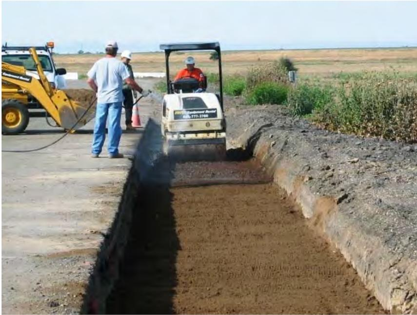
**Figure 2-3. Soil Compaction of Fill Soil in 4 to 6 Inch Lifts**
