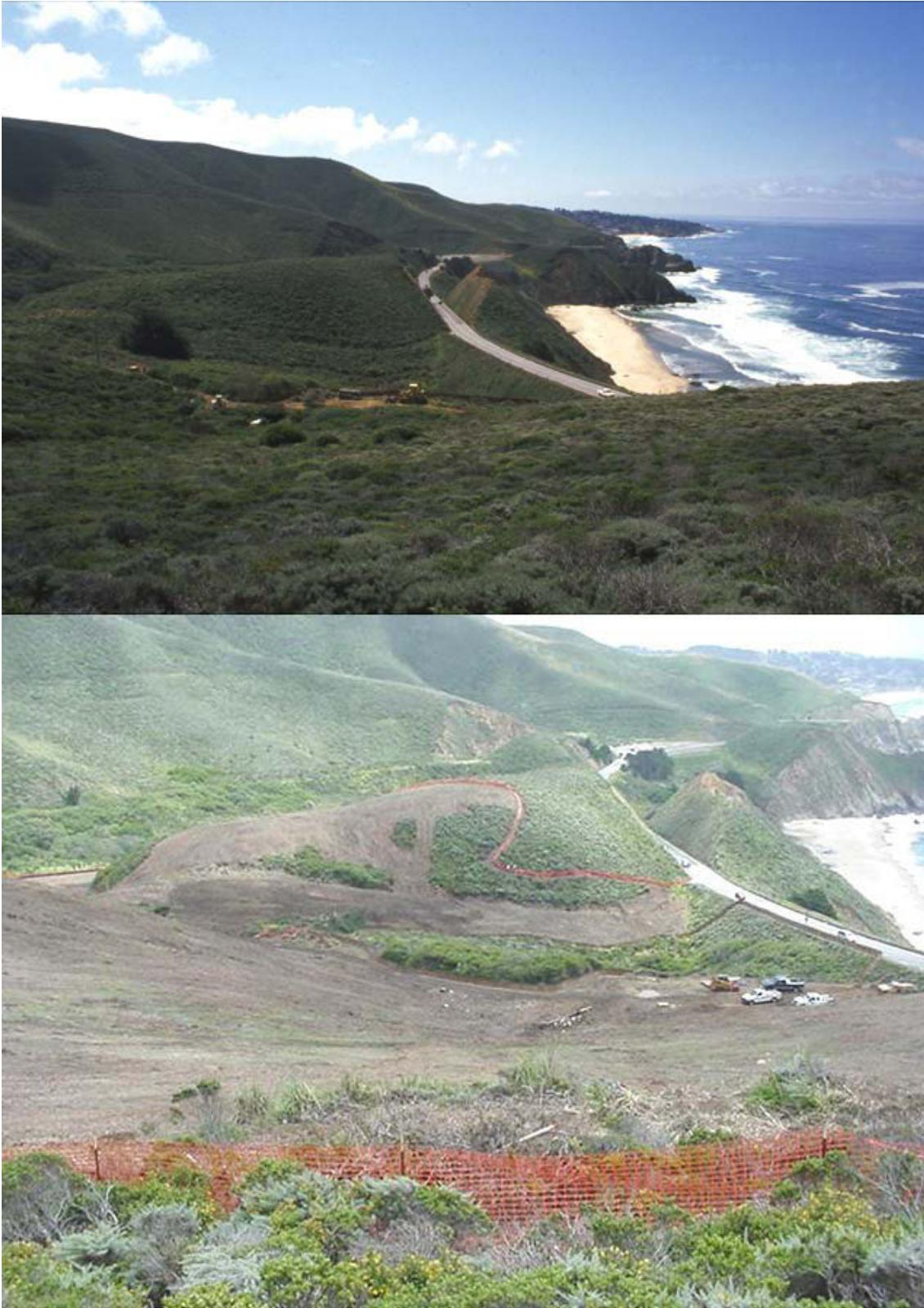
Figure 15. Devil's Slide disposal area before (top) and after clearing and grubbing.
