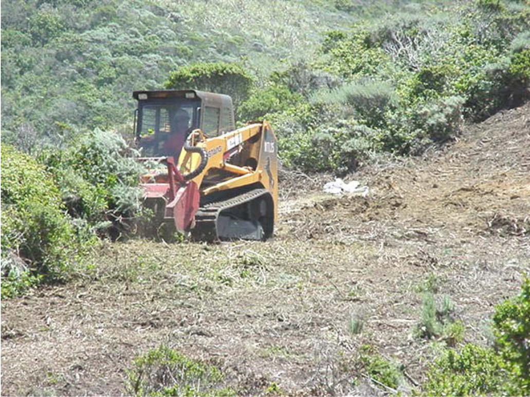
**Figure 14. Clearing and grubbing operation at Devil's Slide to prepare the disposal site.**
