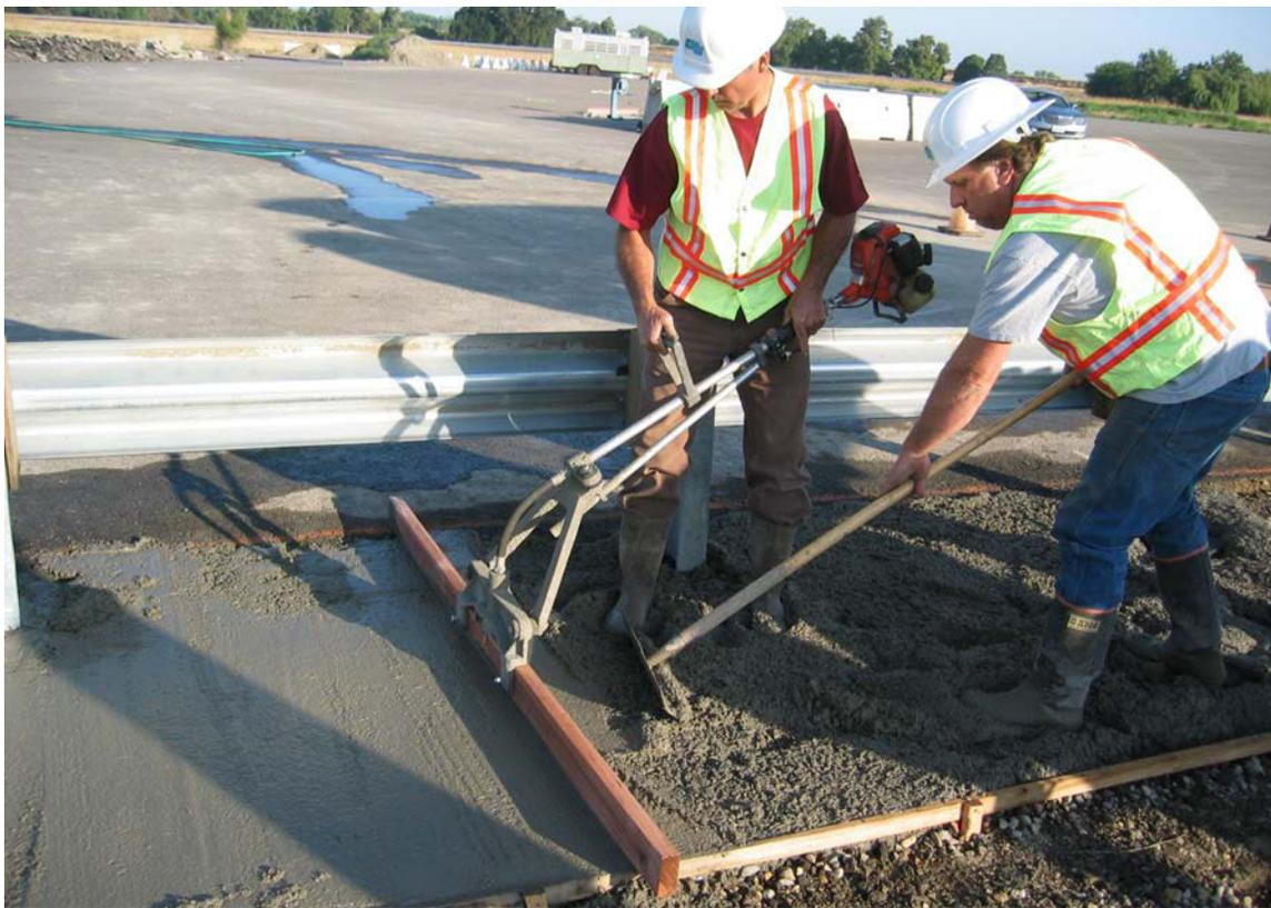
Figure 2-11 – Screeding and Compaction of CRMCrete for Test 658
