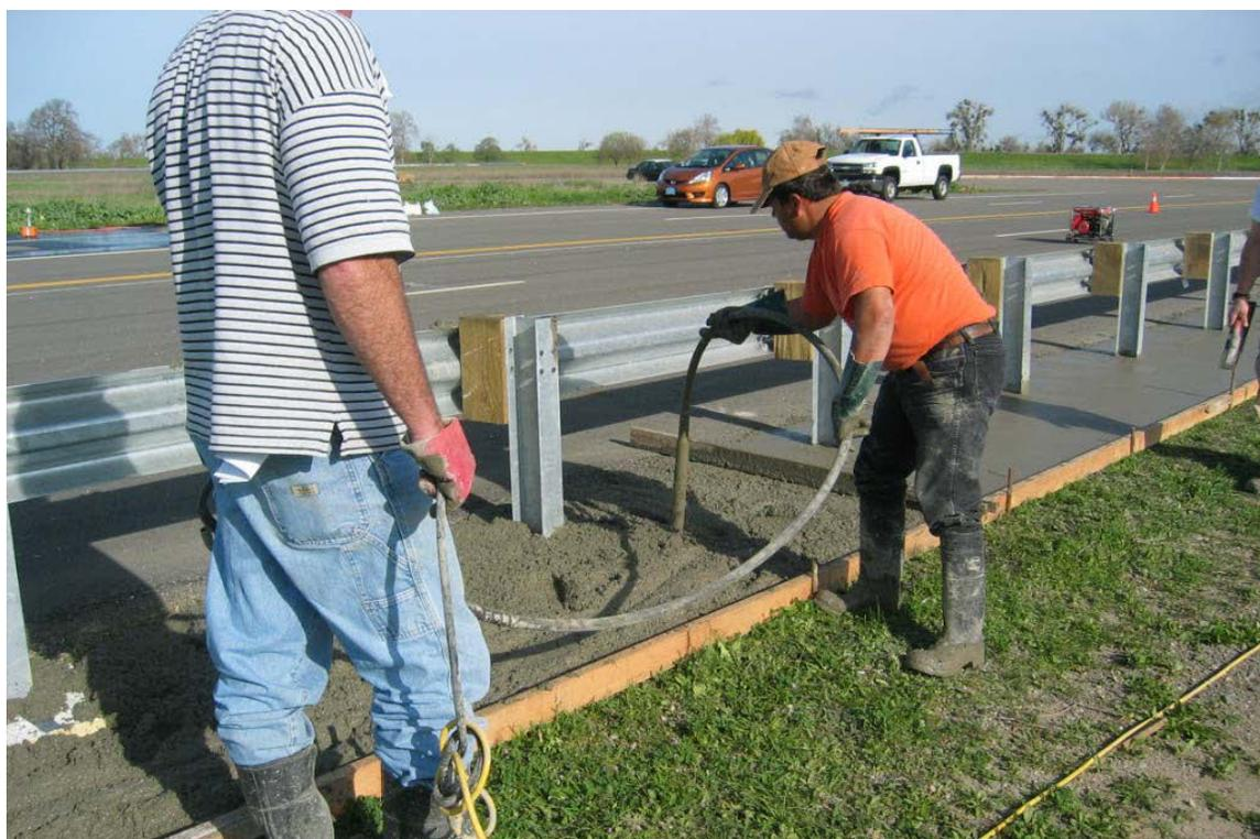
Figure 2-29 – Test 659 Placing of the CRMCrete
