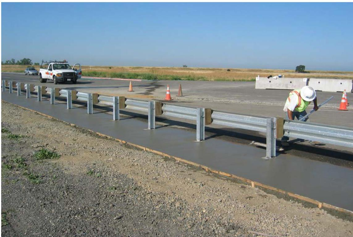
Figure 2-12 – CRMCrete Finishing for Test 658
