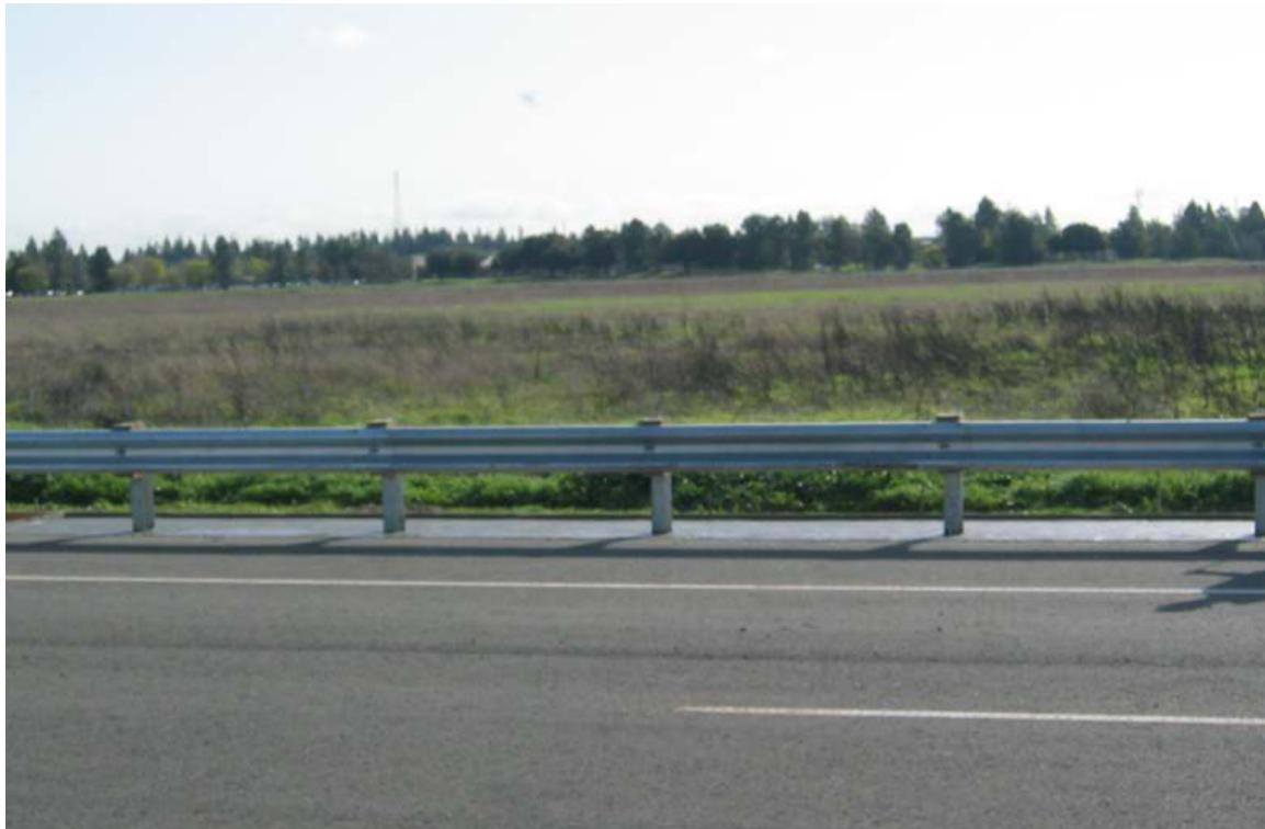
Figure 2-30 – Test 659 Completed Guardrail and CRMCrete Installation
