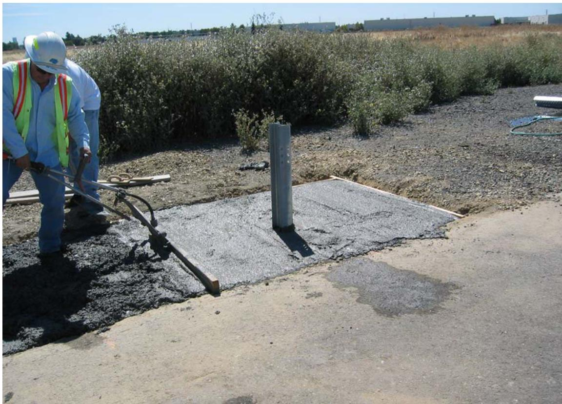
Figure 2-6 – CRMCrete Placement for Bogie Tests
