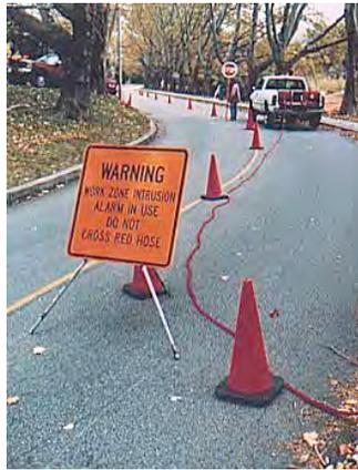
Figure 2. Typical Perimeter System Using Pneumatic Tubes<sup>[3]</sup>
