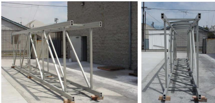
Figure 30 Trial assembly of Snap-fit Truss Structure for this Project
