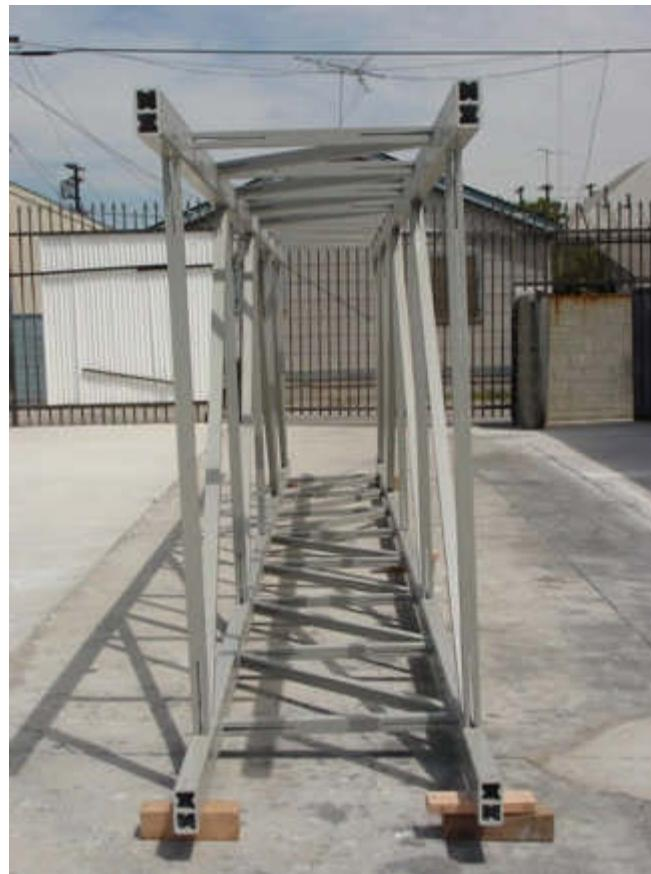
Figure 25 Assembled Overhead Sign Structure
