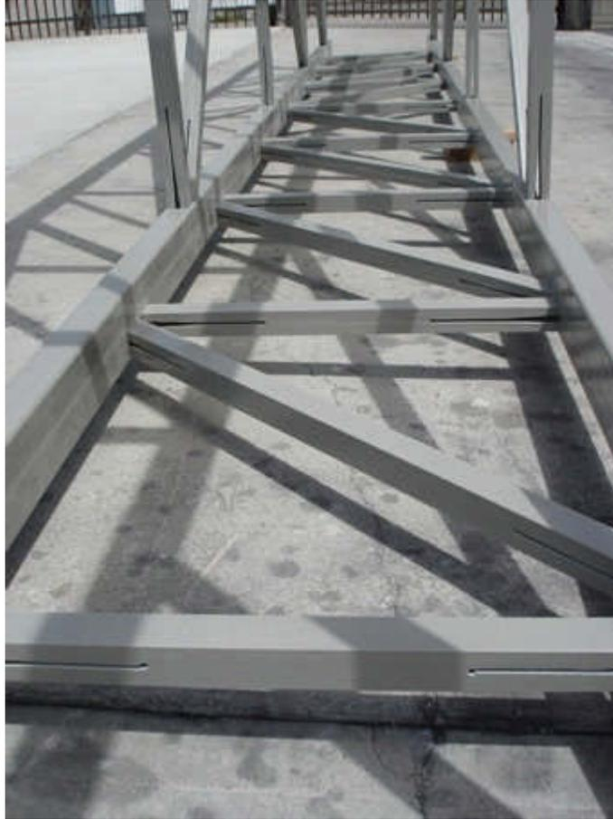
Figure 26 Assembled Overhead Sign Structure
