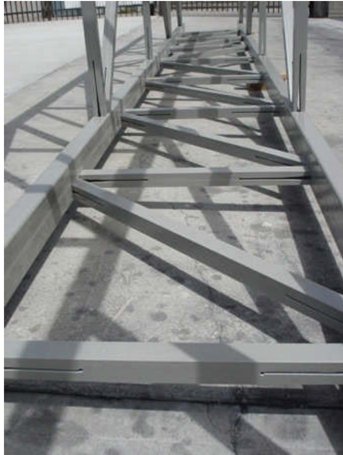
Figure 26 Assembled Overhead Sign Structure
