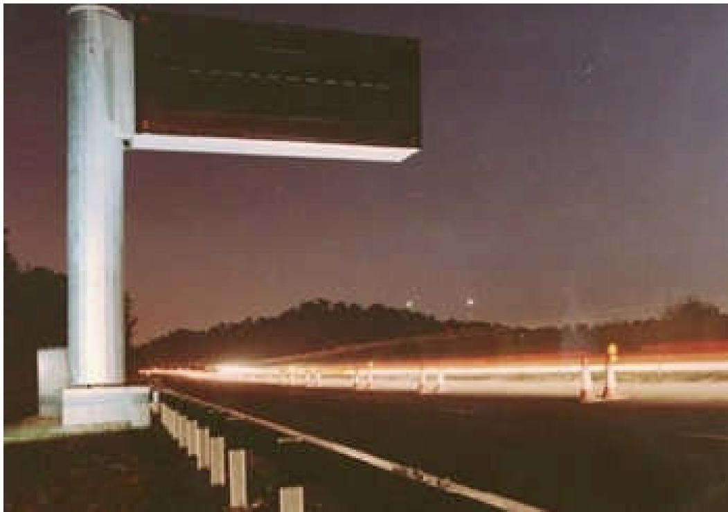
Figure 4 Composite Variable Message Sign Structure with Steel Post
