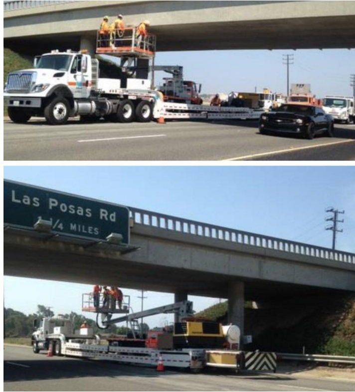
Figure 4.6: Highway sign maintenance & installation (courtesy of district 7).
