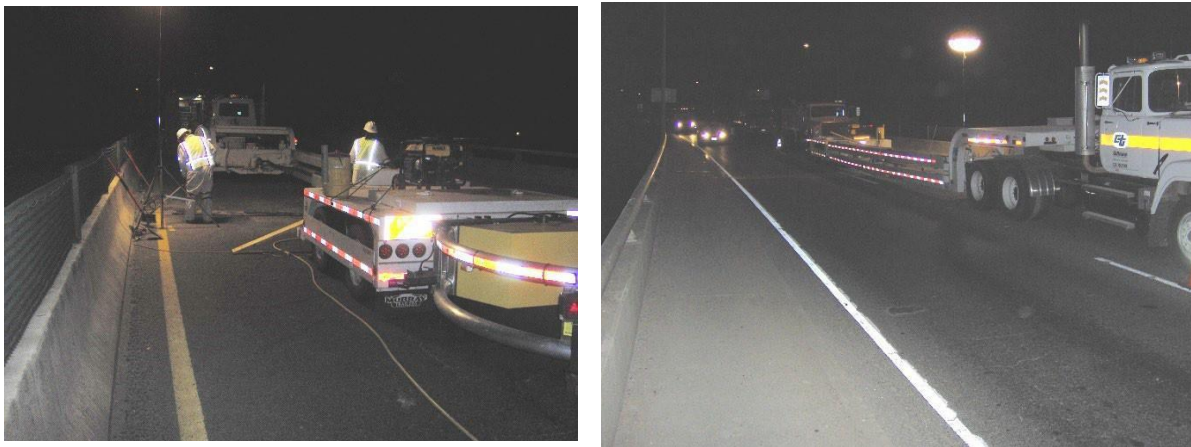
Figure 4.2: Concrete Pour on a bridge deck (Courtesy of District 11).
