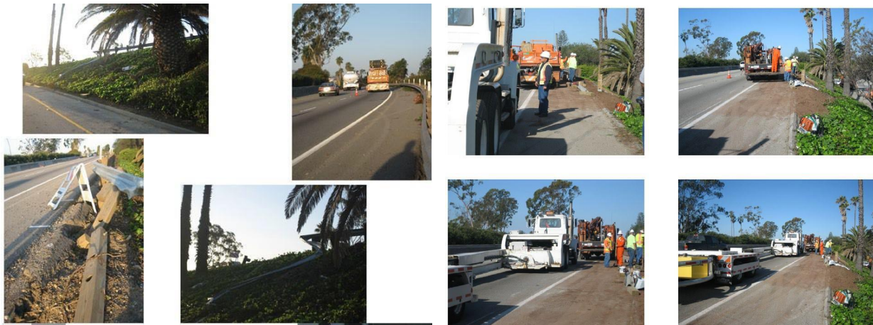
Figure 4.5: Guardrail repair (courtesy of district 5).
