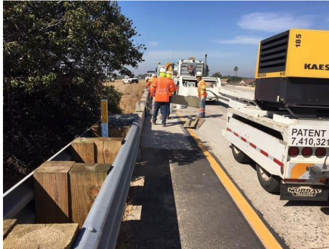
Figure 4.4: Guardrail repair (courtesy of District 11).
