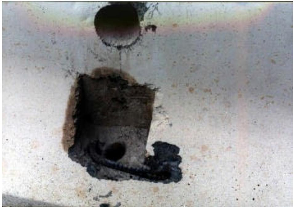
Figure 2-3 - Exposed Rebar
