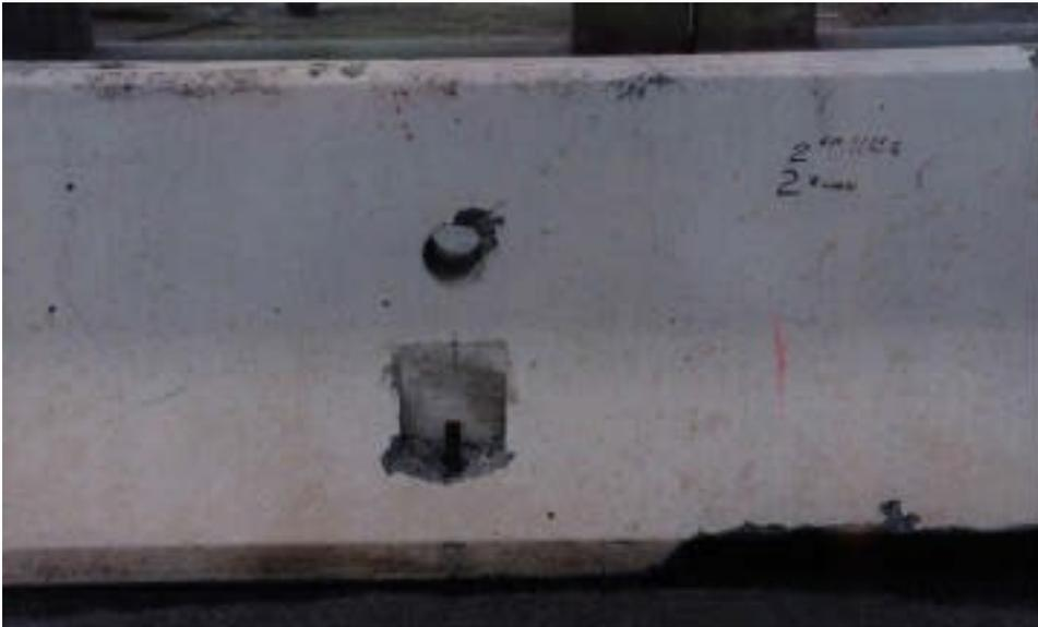
Figure 2-2 - View of Anchor Stake in Barrier
