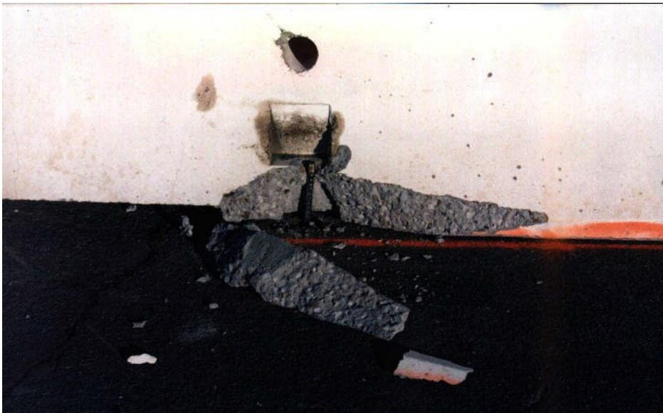
Figure 2-12 - Concrete Spalling At Anchor Stake
