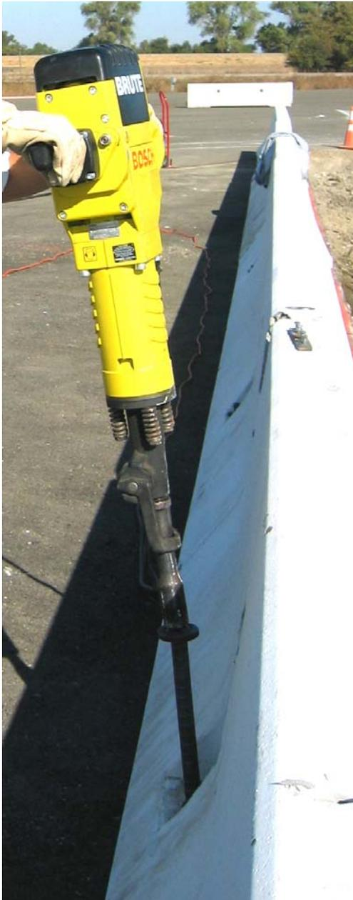
Figure 7-7. Stake Installation
