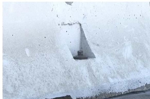
Figure 7-10. Installed Capped Stake
