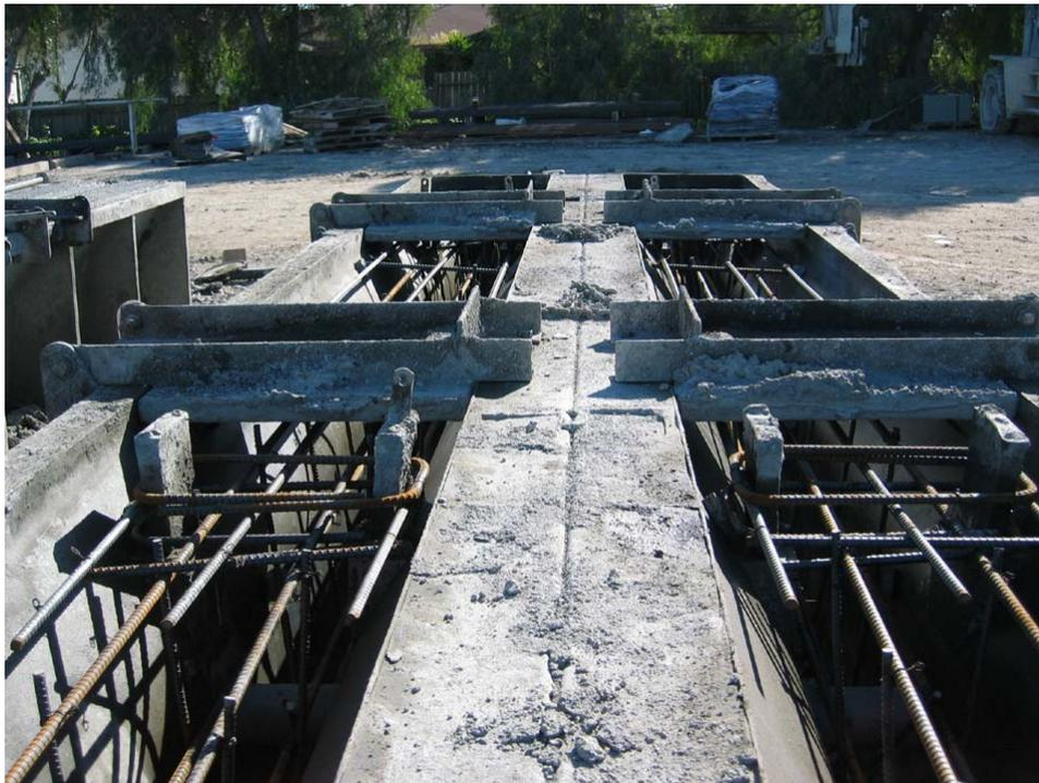
Figure 2-2. K-rail Rebar Placement
