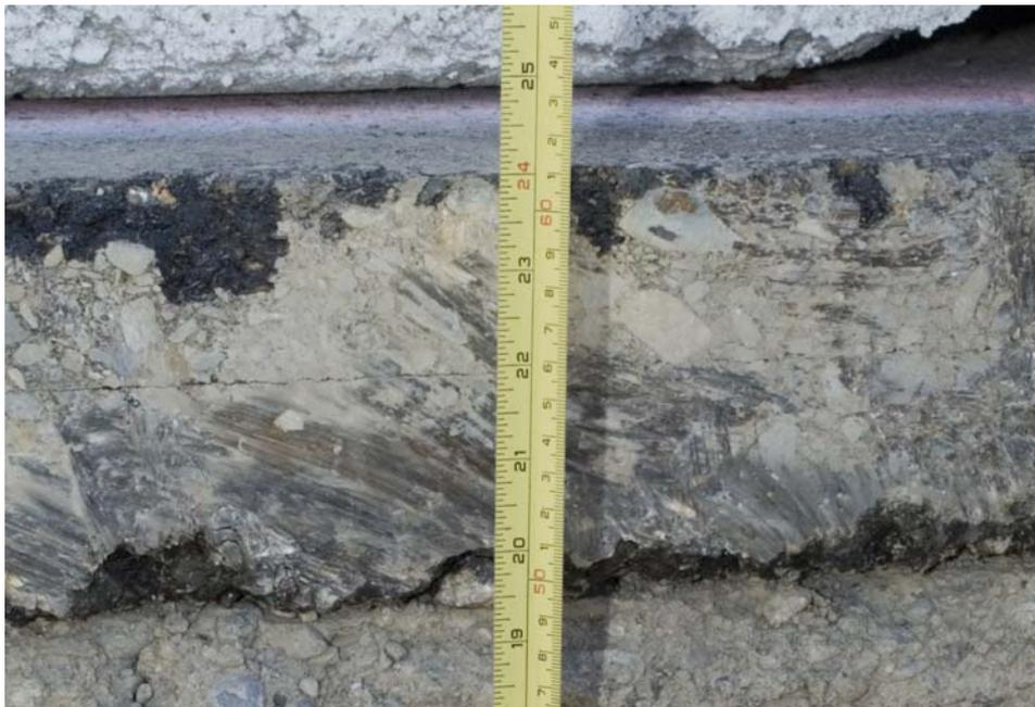
Figure 2-1. Asphalt Concrete Thickness
