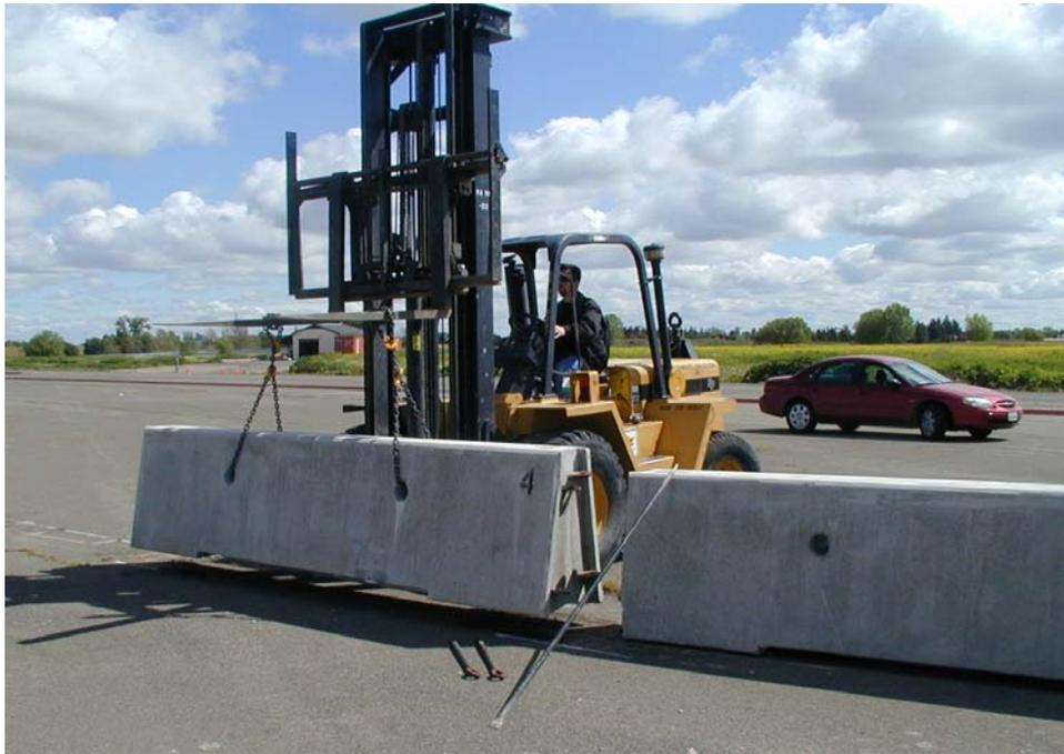
Figure 2-1 – Barrier Placement
