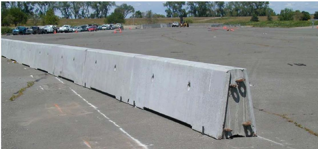
Figure 2-4 – Backside of Completed Barrier with Stakes
