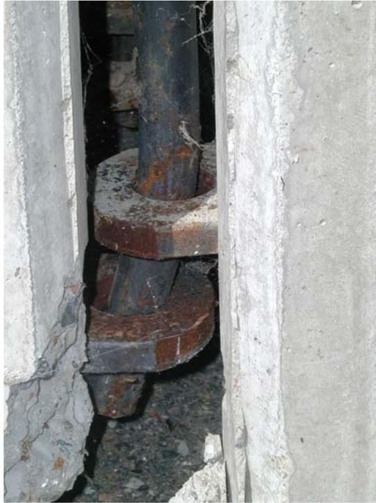
Figure 2-16 – Close-up of Bent Pin at Joint 8-9
