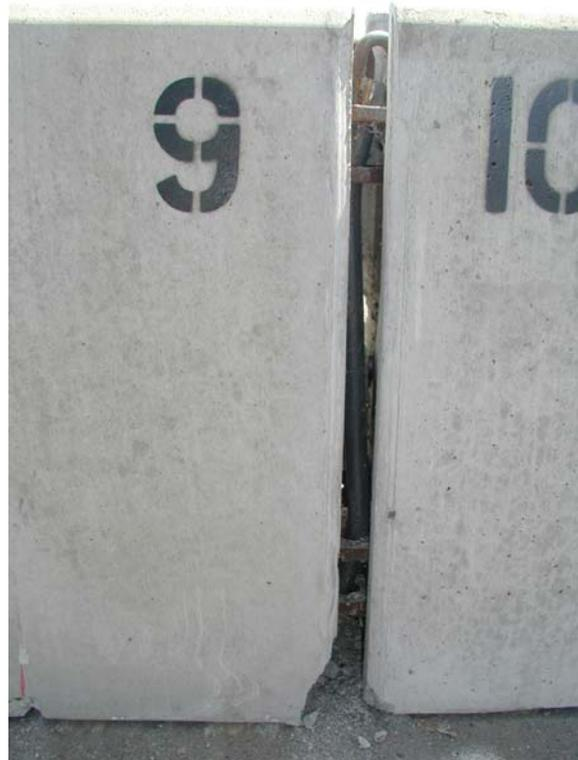
Figure 2-15 – Backside of Joint 8-9 showing Minor Concrete Spalling and Bent Pin (mislabeled)
