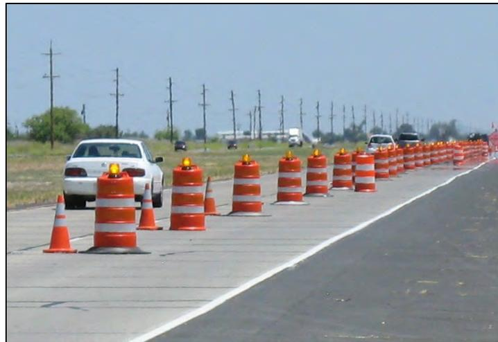
**Figure 6: Warning Light Brightness – WTI Photo**
