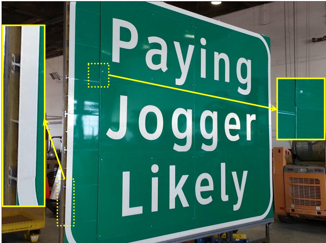
**Figure 3.3. Overhead Guide Sign Construction.**
