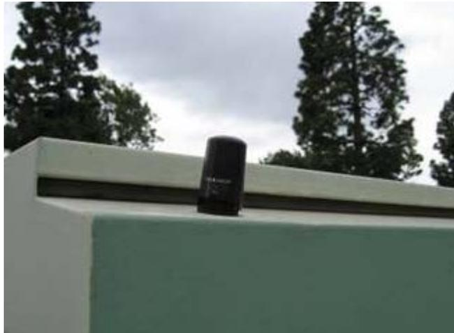
**Figure 4-16: Typical WLAN Client Antenna Installation**
