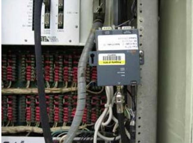
**Figure 4-15: Typical WLAN Client Intersection Cabinet Installation**
