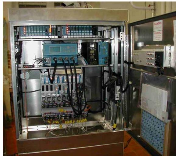
The traffic controller cabinet shown above includes a NEMA Econolite ASC/2 controller.
