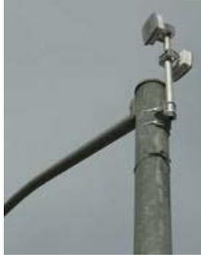
**Figure 4-13: Typical WLAN Bridge/AP Equipment Installation**
