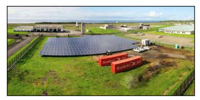
1.75MW, and another 500+kW of roof-mounted PV's in place funded by the American Recovery and Reinvestment Act (ARRA). The PV farms which were installed after the tsunami in April 2012 above the inundation area of the tsunami.<sup>94</sup>
