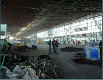
Nonstructural damage included damage to more than 80% of the ceilings throughout the airport, breakage of fire sprinkler pipe with extensive water damage, collapse of hot water piping, partition damage, extensive damage to retail space, damage to light fixtures, collapse of most suspended air handling units, damage to cable trays, damage
