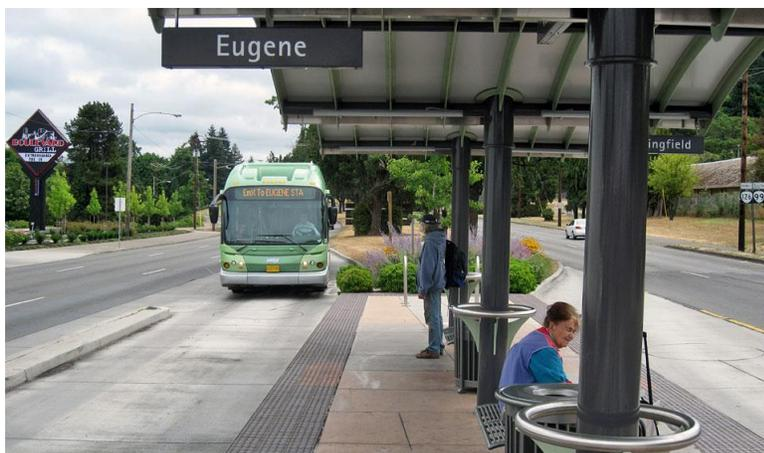
**Figure 4:** An Emerald Express bus pulls into a station in the median of Franklin Boulevard in Eugene, Oregon. While the Eugene-Springfield BRT required converting general-purpose lanes, previous traffic conditions were so relatively light that adding BRT lanes caused little or no congestion in the remaining lanes. Source: Darrell Clarke, 2008
