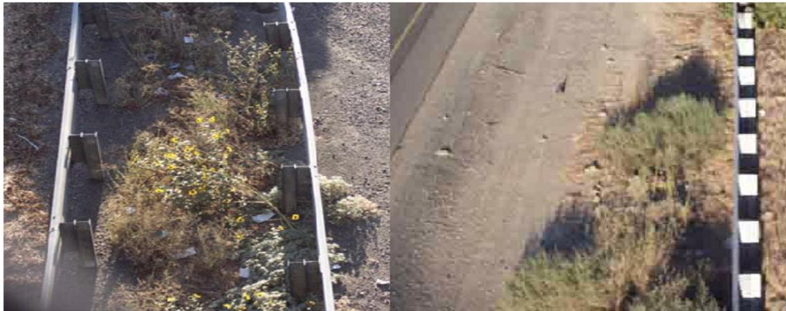
*Figure 4.2 Vegetation and debris in between and around guard rails.*
