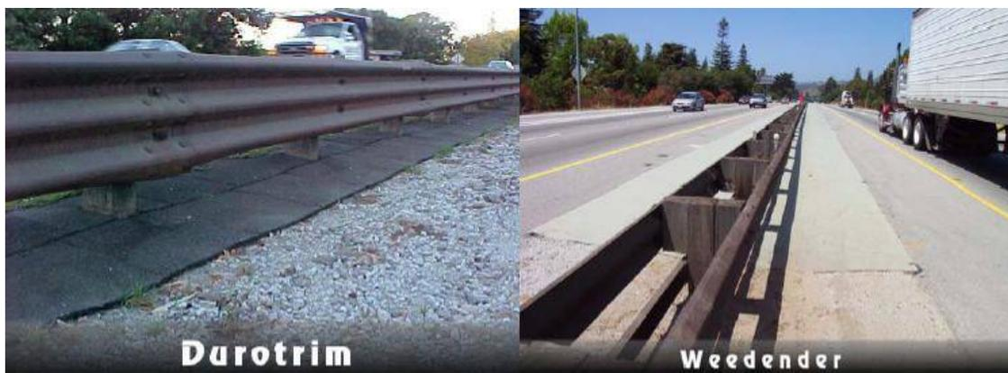
*Figure 2.2 Different weed mat products tested on California highways*
