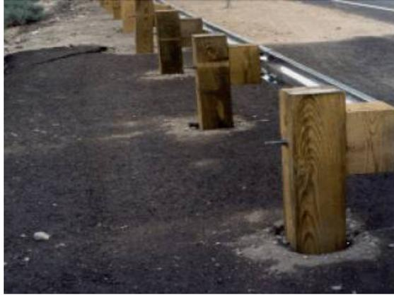
*Figure 2.11 Asphalt concrete hardscape*
