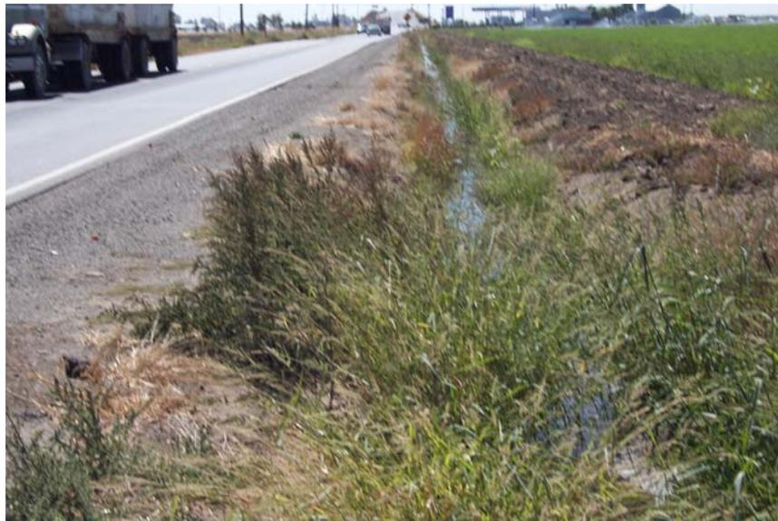
*Figure 1.5 V-type Ditch With Irrigation Water*
