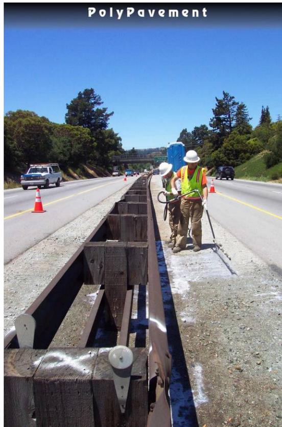
*Figure 2.1 Caltrans workers applying PolyPavement weed barrier*
