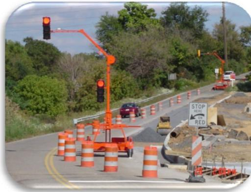
**Figure 11. Portable Traffic Signal.**
