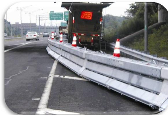
**Figure 9. Example of Steel Barrier.**
