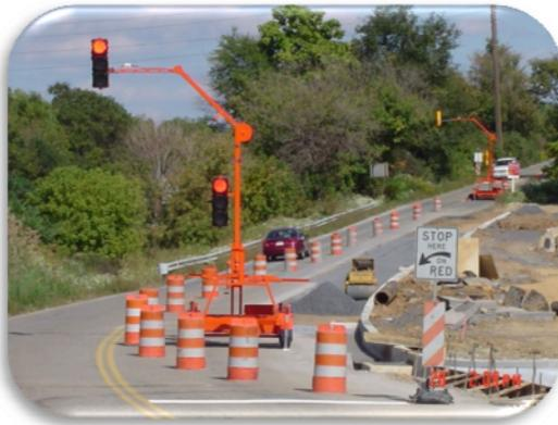
Portable traffic signals are traffic signals mounted on trailers that can be used to control the right-of-way in a work zone. Communications between the signals are provided by hard wiring, radio frequency transceiver, or by preset timing. Thus, portable traffic signals can actually replace flaggers; thereby, removing flaggers from direct exposure to approaching traffic and allowing flaggers to perform other critical work tasks.
