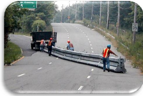
Some steel barrier designs include retractable wheels that can be lowered so that the steel sections can be moved by hand laterally across travel lanes as needed to create protected work spaces. Other designs include wheels and vehicle attachments that allow the barrier to be moved along with the work activity as it progress down the roadway.
