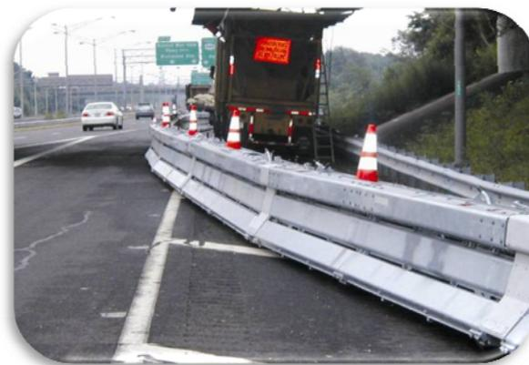
**Figure 9. Example of Steel Barrier.**
