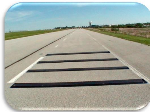
**Figure 5. Portable Plastic Rumble Strips.**
