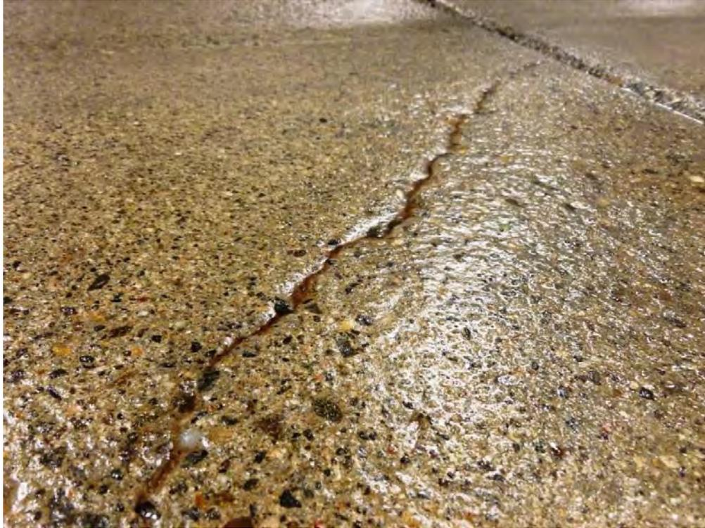
**Figure 34: Close-up of methacrylate-filled crack.**
