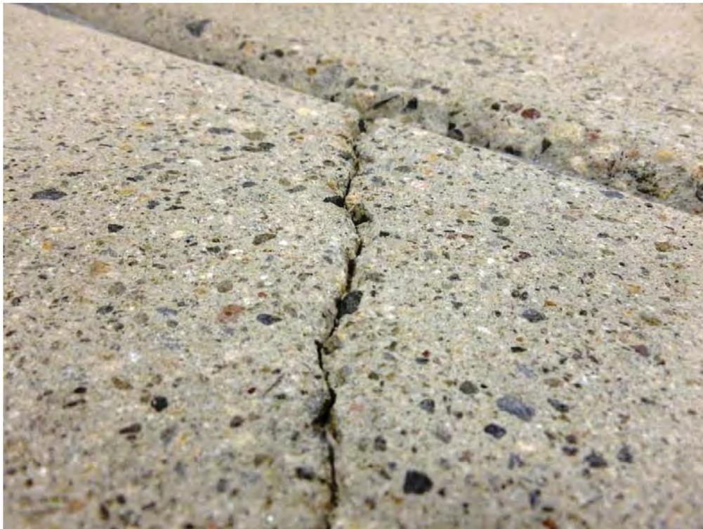
**Figure 32: Crack in deck surface after shot blasting.**
