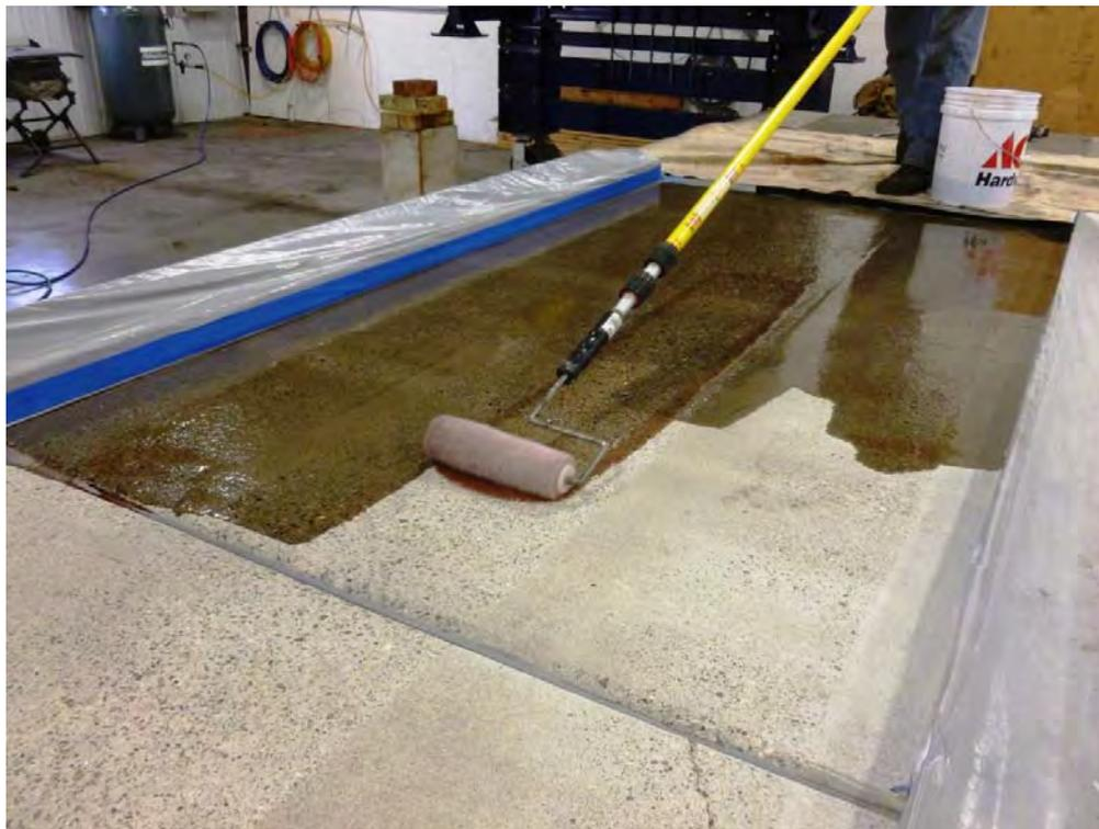
**Figure 33: Application of HMWM surface treatment.**
