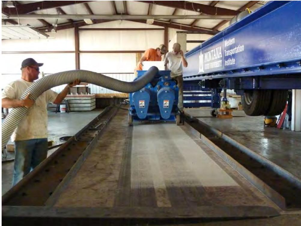
**Figure 30: Shot blasting the deck panels in preparation for the HMWM application.**
