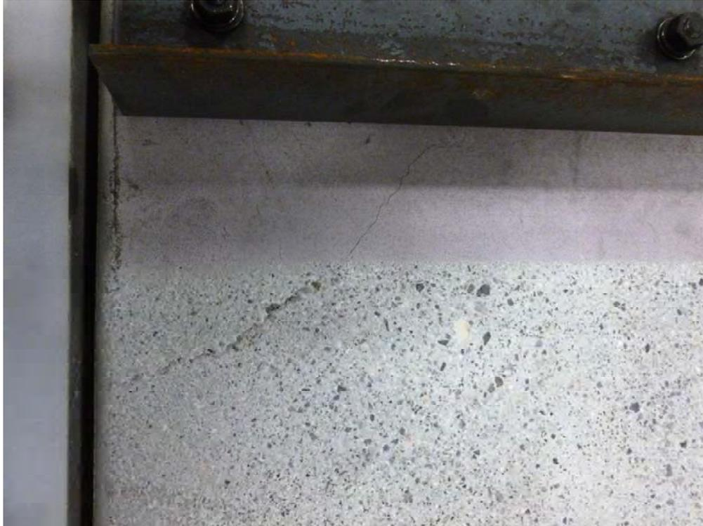
**Figure 31: Concrete surface before and after shot blasting.**
