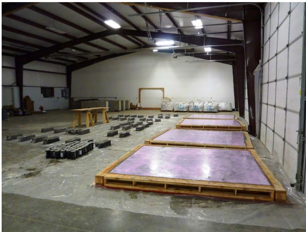
**Figure 13: Finished slabs with concrete curing compound on surface.**
