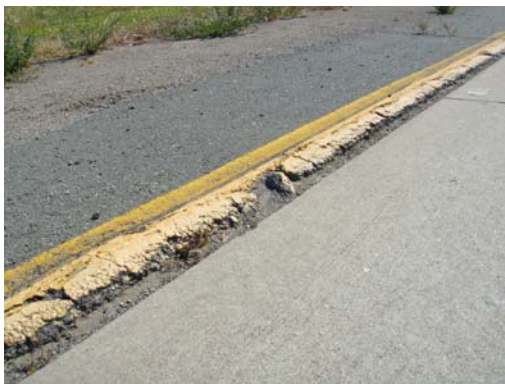
Figure 10. Shoulder Crack Lipping – Hwy 160
