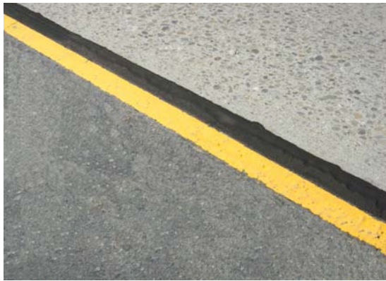
Figure 13. Effective Joint Seal - Hwy 160
