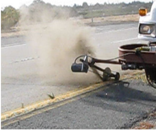
Figure 16. Sealzall Crack Cleaning Attachments – Hwy 160
