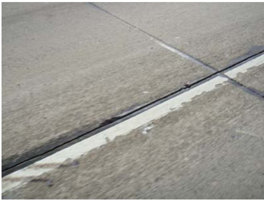
Figure 8. Failed In-lane Seal between Lanes 1-2
