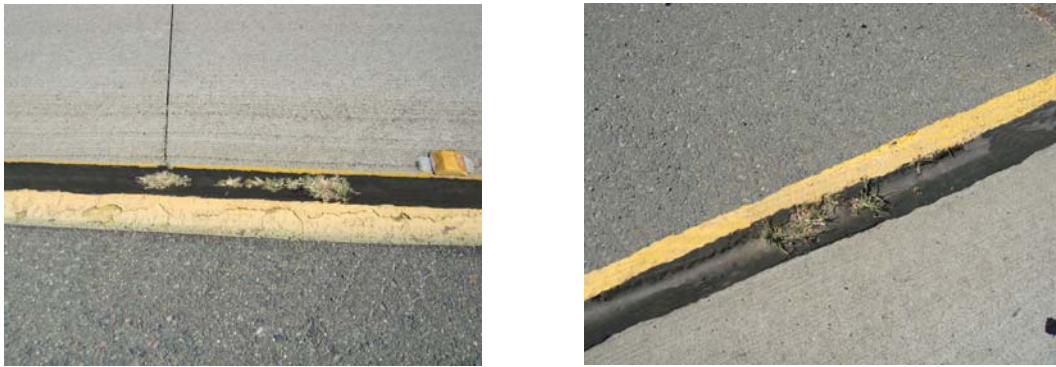
Figure 12. Vegetation in Seal after only 6 Months - Hwy 160
