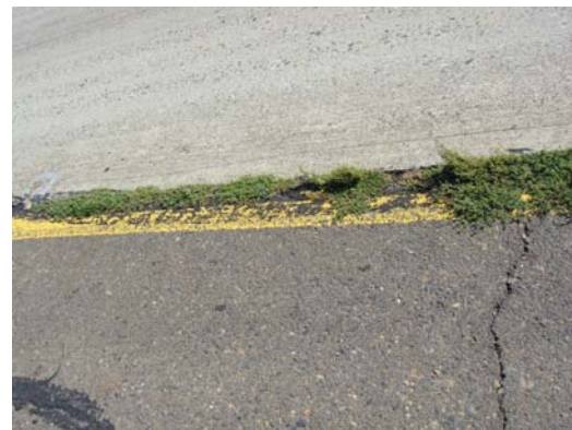
Figure 9. Failed Longitudinal Edge Joint Seal
