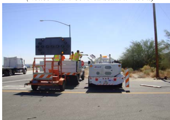
Figure 5. Loading Sealant Blocks - Hwy 86
