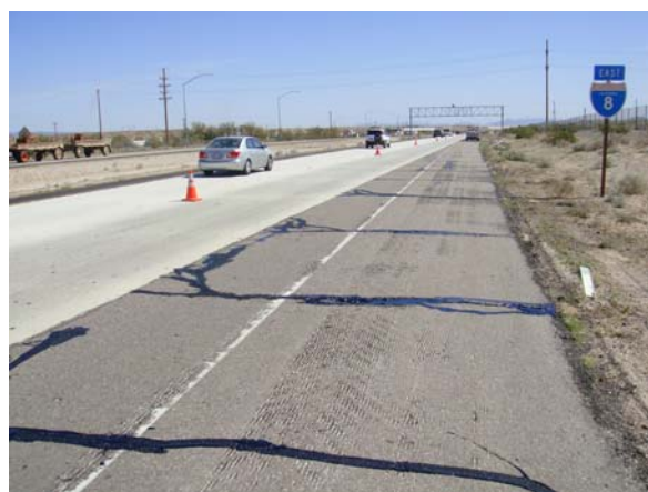
Figure 6. Merge Lane Manual Sealing - Hwy 8
