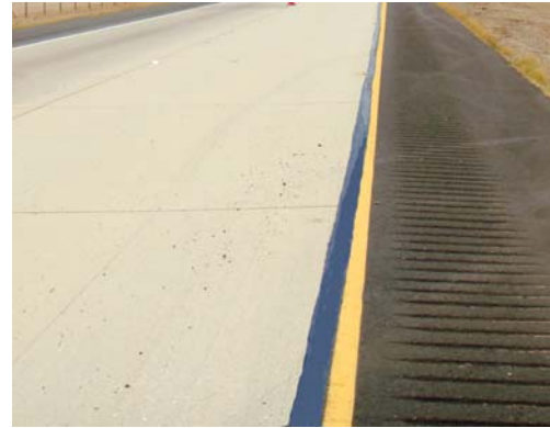
Figure 14. Effective Joint Seal - Interstate 8
