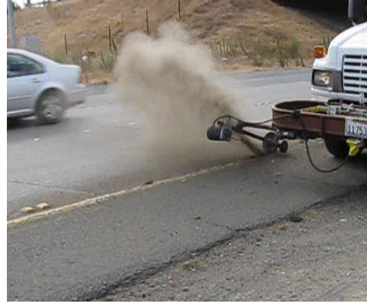
Figure 16. Sealzall Crack Cleaning Attachments – Hwy 160
