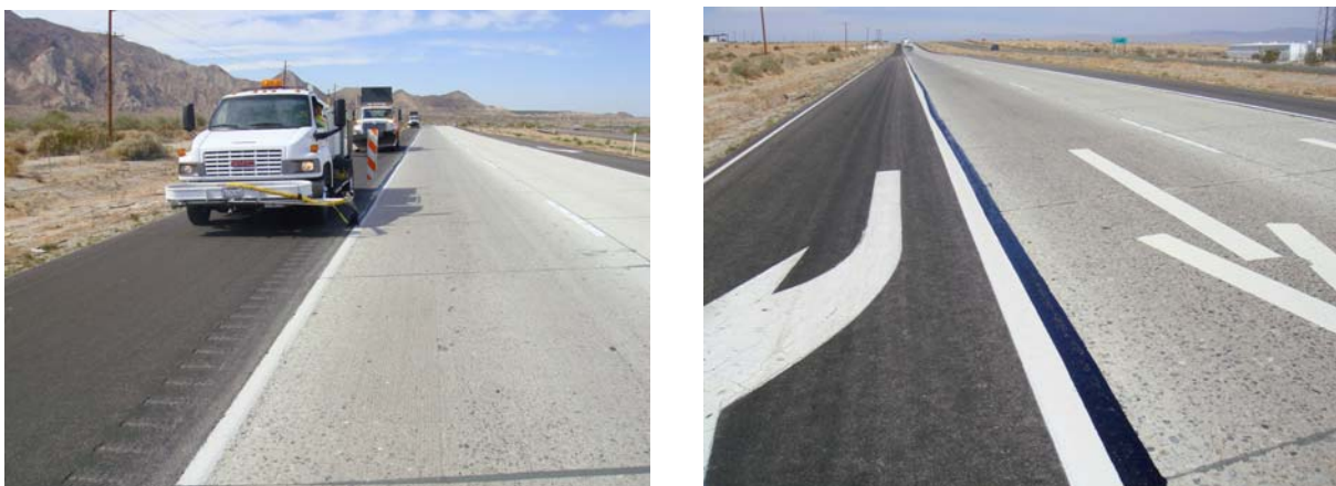
Figure 3. Longitudinal Sealing Highway Shoulder Joint Sealing Operation - Hwy 86
