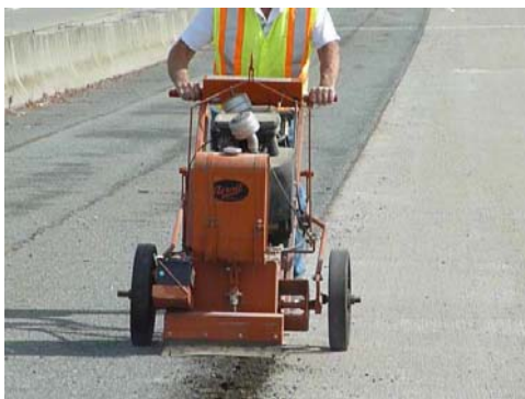
Figure 17. Joint Routing - Interstate 380
