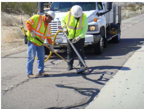
Figure 6. Merge Lane Manual Sealing - Hwy 8
