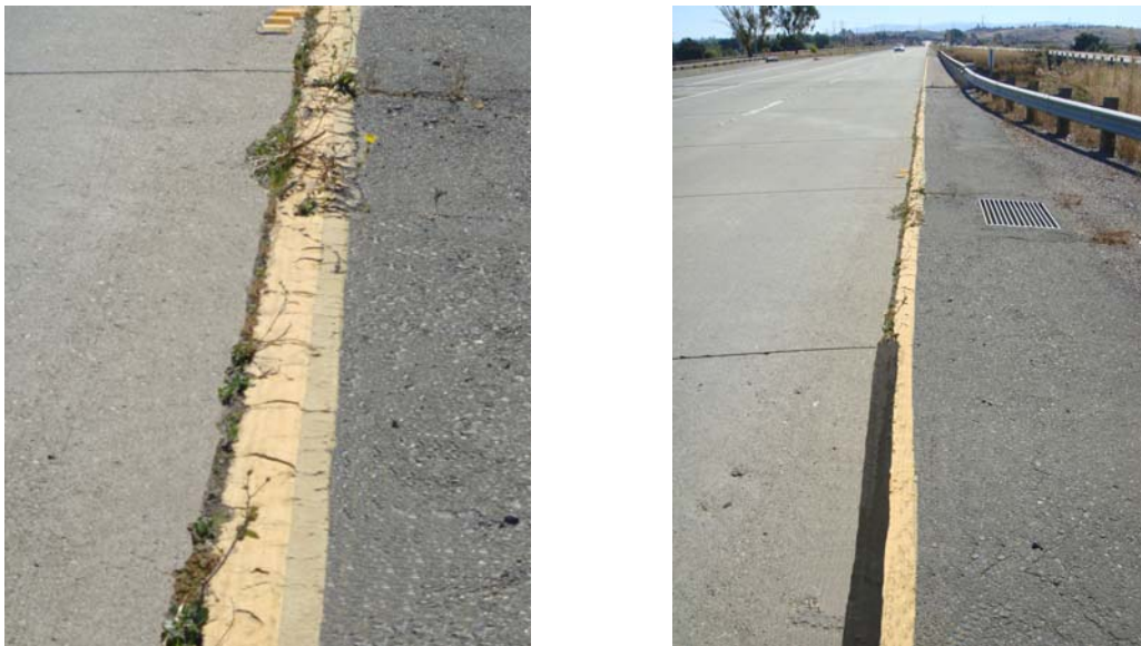
Figure 7. Typical Unsealed Longitudinal Joint and Same Joint Sealed with Proper Cleaning
