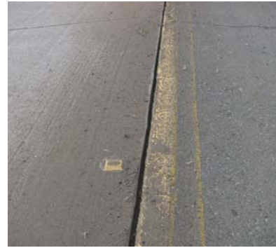
Figure 22. One Pass Routed Joint
