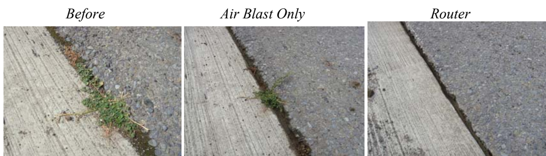
Figure 15. Crack Cleaning Test - Interstate 380
