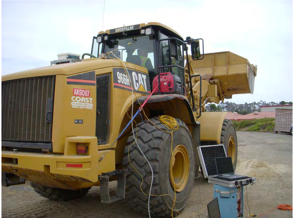
Figure 4. Installation of the Generator and integrated PM Measurement System
