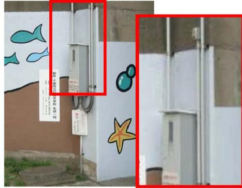
**Figure 2.32 No gaps between A1 abutment and upstream side retaining wall (PWRI 2011)**
