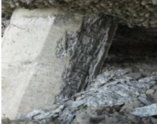
**Figure 2.10 Plastic hinging in abutment piles of Bridge Street Bridge (Palermo et al. 2011)**
