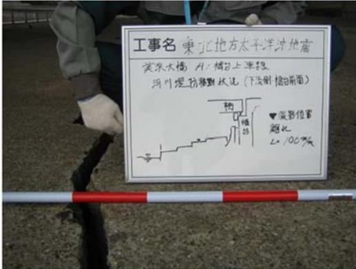
Figure 2.26 Cracks on the sea bank
