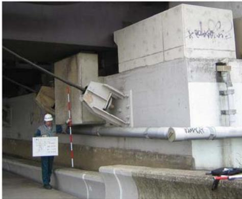
Figure 2.22 Ground settlement at the face of A1 abutment H=630mm (Chiba city 2011)
