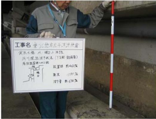
Figure 2.20 Ground settlement at the face of A1 abutment H=(Chiba city 2011)
