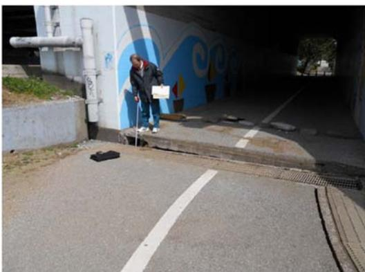
Figure 2.18 Ground settlement at the side of A1 abutment (Chiba city 2011)
