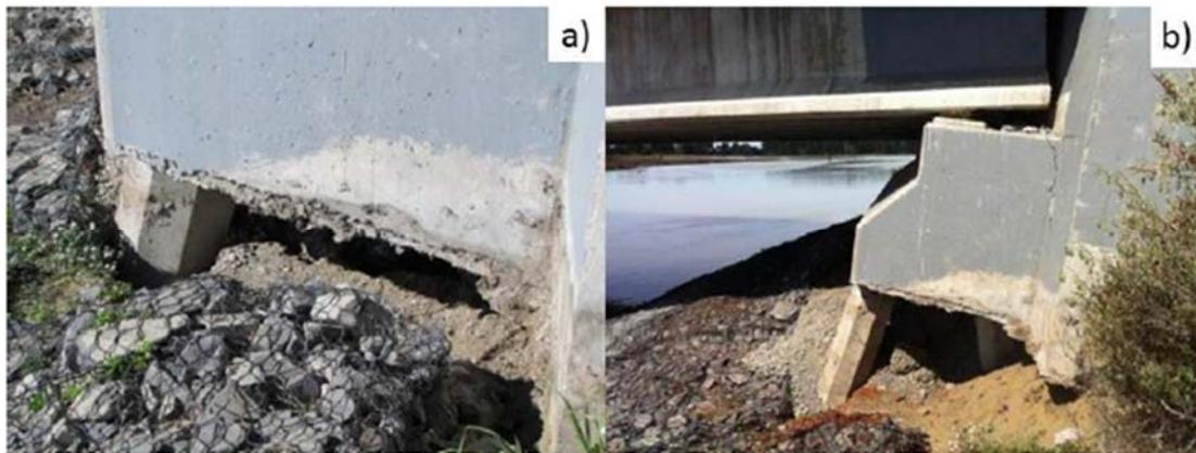
**Figure 2.11 Comparison of the displacement of slope in front of western abutment following, a) Darfield event, b) Christchurch event (NZ-GEER 2011)**
