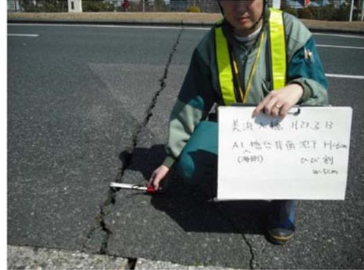
Figure 2.27 Cracks on the A1 abutment
