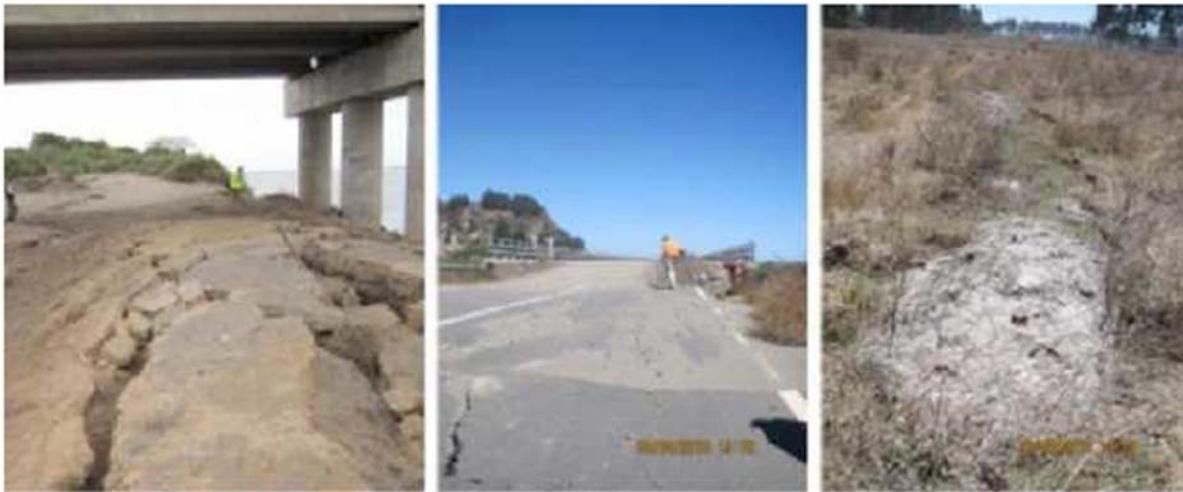
**Figure 2.4 Mataquito bridge: (a) Lateral spreading on the south end of the bridge, S35.050712° W72.162258°; (b) approach fill settlement at the north abutment of the bridge (70 cm offset at the bridge deck), S35.050712° W72.162258°; (c) sand boils at the north end, S35.051961° W72.163217° (Ledezma et al. 2012)**
