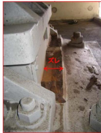
Figure 2.30 Displacement of the bearing of A1 abutment (Chiba city 2011)
