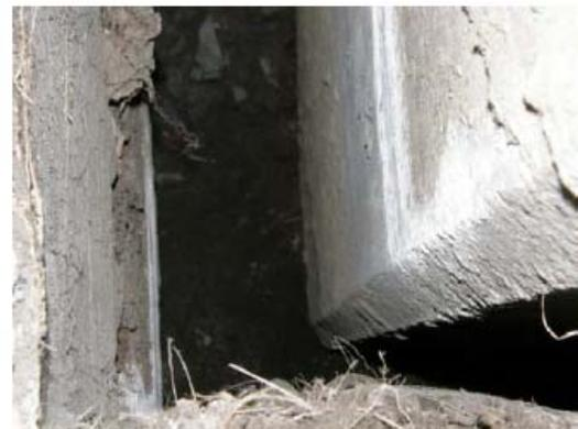
Figure 2.23 Gap at the face of A1 abutment (Chiba city 2011)
