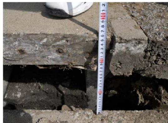
Figure 2.19 Ground settlement at the side of A1 abutment (H=260mm) (Chiba city 2011)
