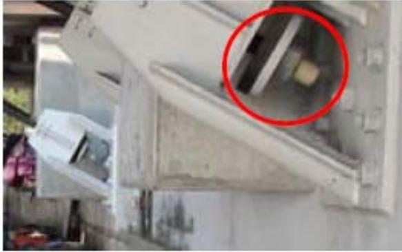
**Figure 2.31 Loosed bridge fall prevention device (PWRI 2011)**
