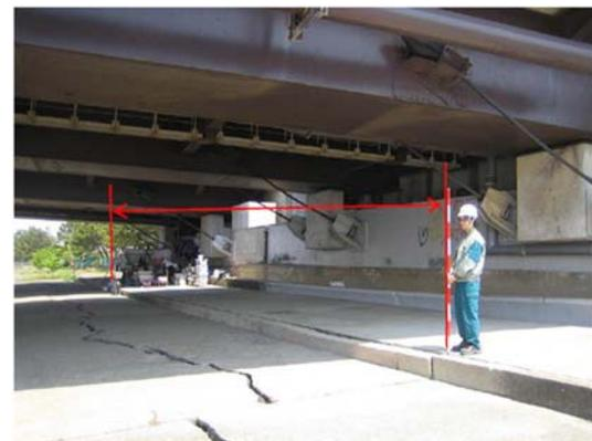
Figure 2.25 Cracks on the sea bank in front of the A1 abutment (Chiba city 2011)
