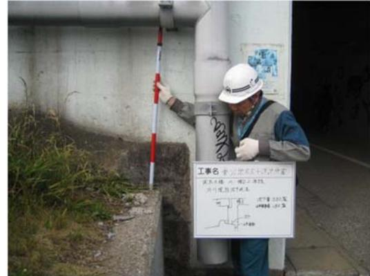
Figure 2.21 Ground displacement (L=180mm) and settlement (H=330mm) near A1 abutment (Chiba city 2011)
