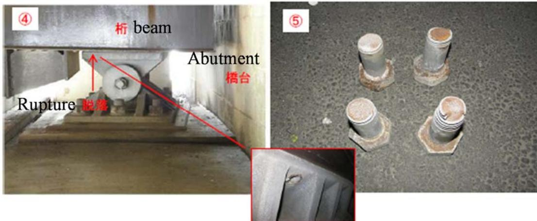
Figure 2.17 Ruptured bolts of A2 abutment (Chiba city 2011)
