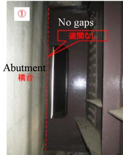
Figure 2.16 No gaps between the deck and A2 abutment (Chiba city 2011)
