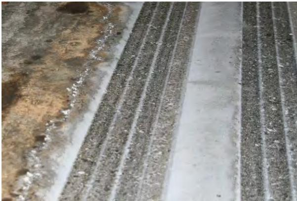
**Figure 4.28: 605FD: Crystallized salt on edges of wheelpaths during early testing.**
