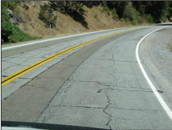
**Figure 2.1: Alligator B and C cracking and digouts.**
