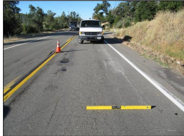
**Figure 2.2: Wheelpath cracking, patching, pumping.**
