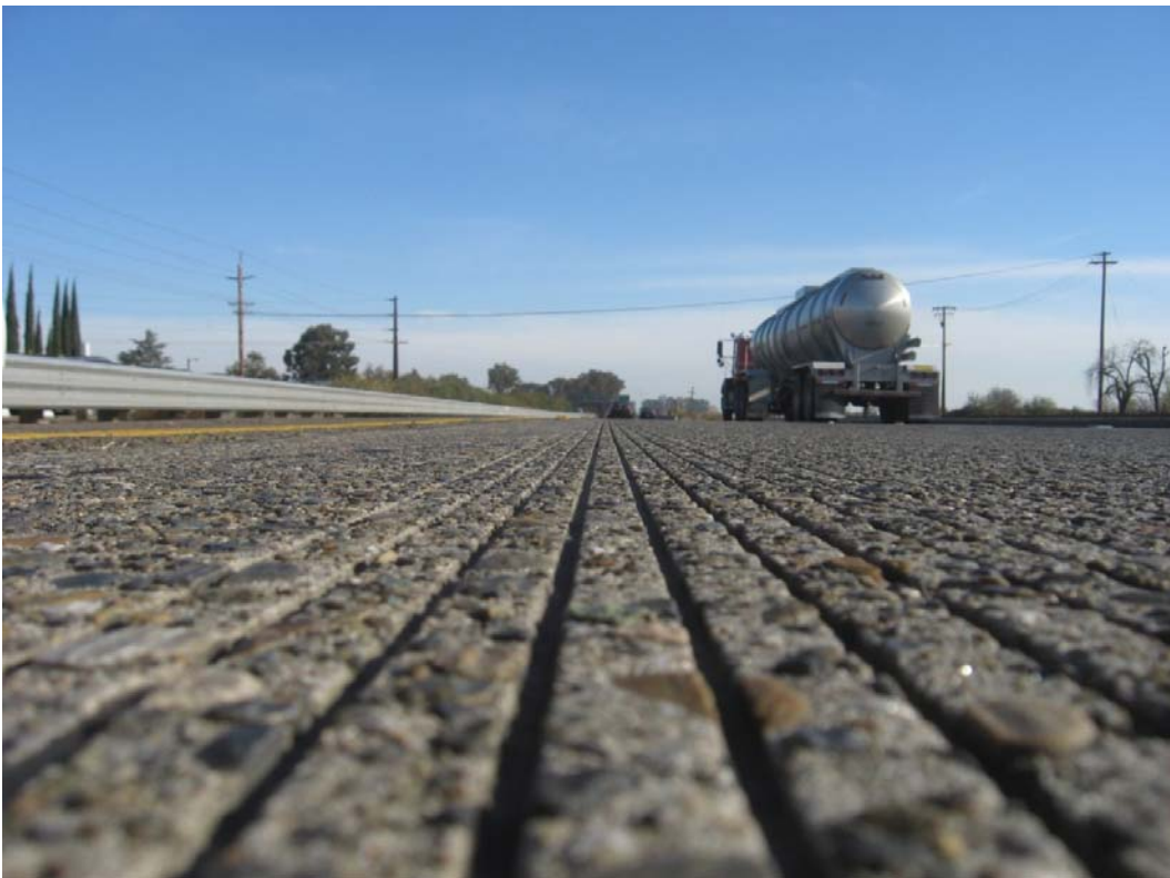
Figure A.6: Diamond grooved, OBSI=105.6 dB(A) (Section QP-153.2).
