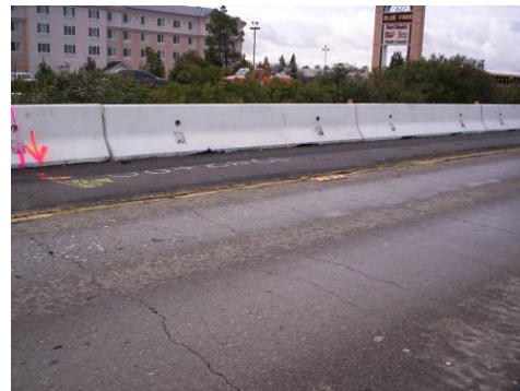
Transverse cracks detail
