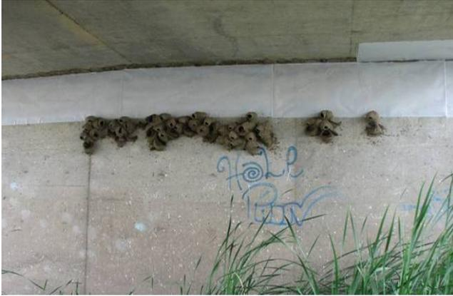
Figure 16. Completed nests below the bottom edge of PTFE treatments on a pier wall.
