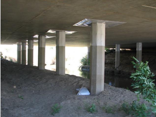
Figure 3. Highway structures with PTFE surface modification.
