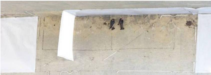
Figure 15. PTFE sheets detaching from the highway structure surfaces and cliff swallows building nests.
