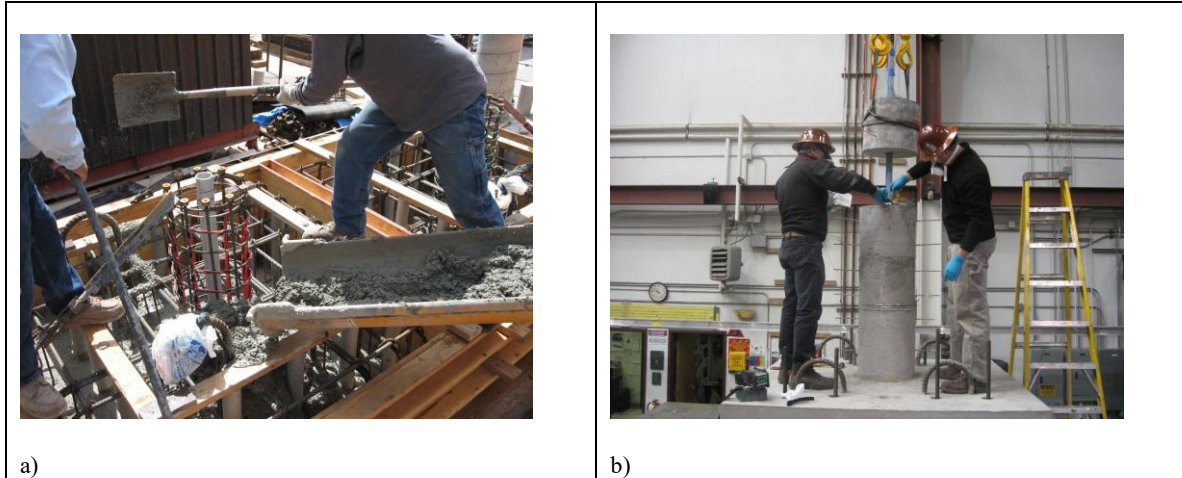
Fig. 4- Footing and the Base Segment steel Cages, b) Assembling Process in Segmental Columns
