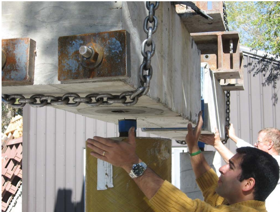
Fig. 2-77. Cap Beam Installation
