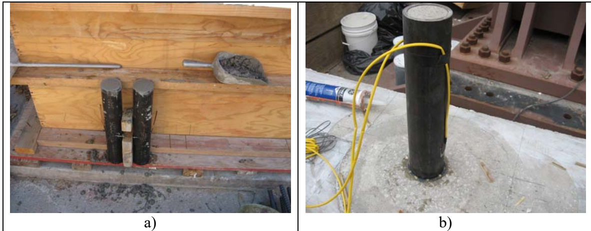
Fig. 2-68. Steel Pipe-Pin, a) Filled with Concrete, b) Sat on the Cap Beam
