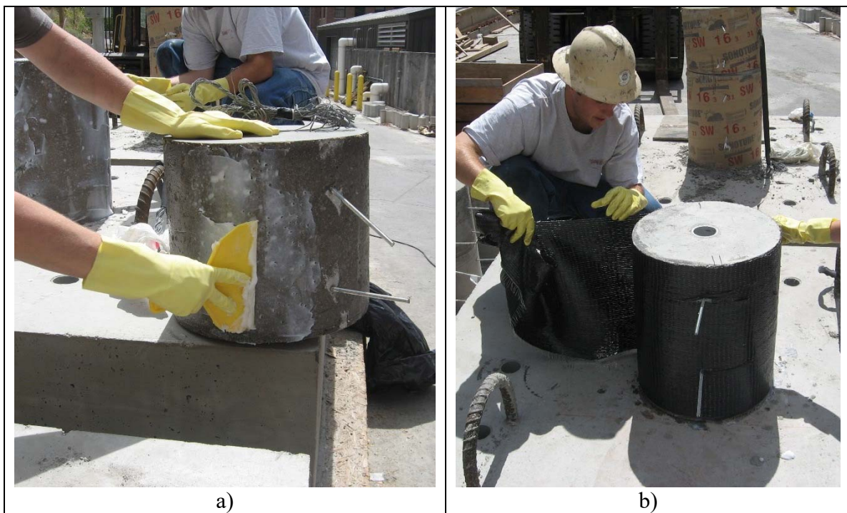
Fig. 2-40. a) Preparing the Surface, b) FRP Wrapping
