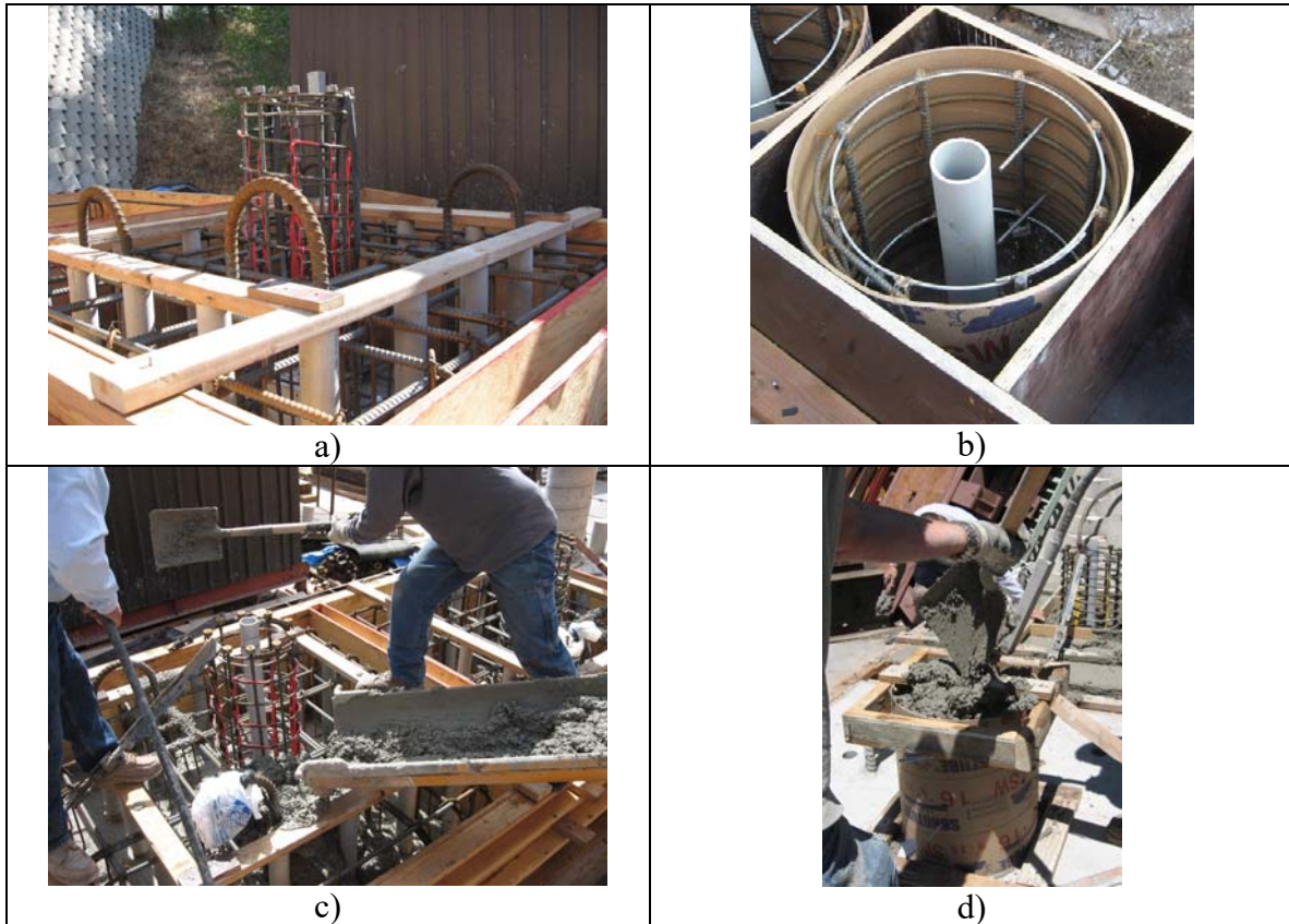
Fig. 2-17. a) Base Segment before Concrete Casting, b) Typical Segment Cage, c) Casting the Footing, d) Casting the Base Segment
