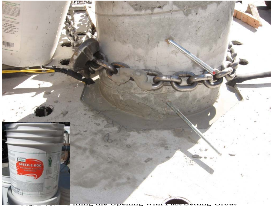
Fig. 2-78. Filling the opening with Fast Setting Grout
