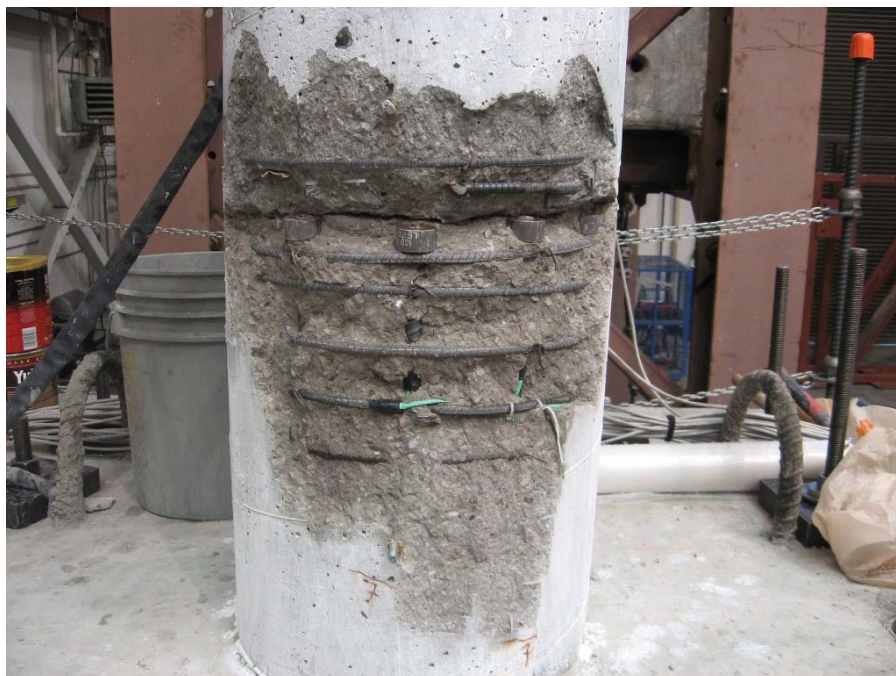
Fig. 2-52. SC-2R Repair Process, Removing Loose Concrete
