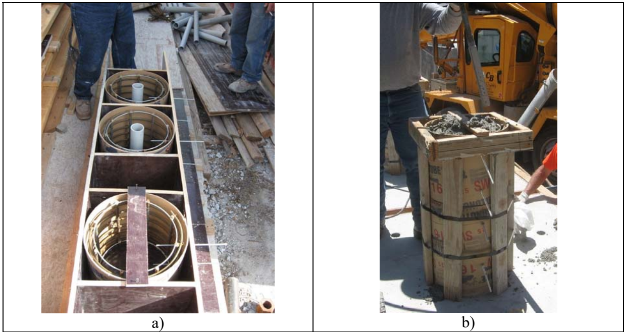
Fig. 2-39. a) Typical Segment Column Cages, b) Constructing the Second Segment with Match Cast Method
