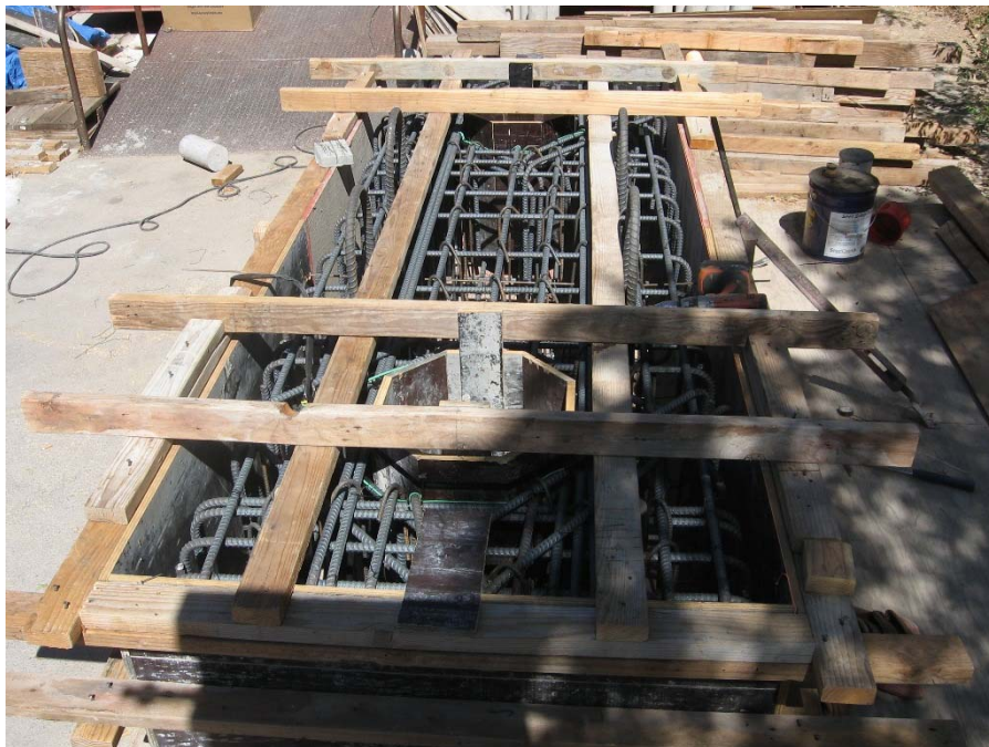
Fig. 2-71. PEFB Footing before Casting of Concrete
