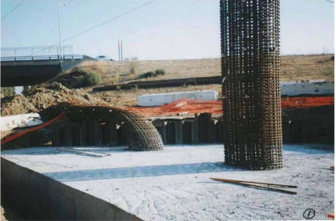
**Figure 1.1: Collapse of Bridge Column Rebar Cage in Milpitas, CA**
