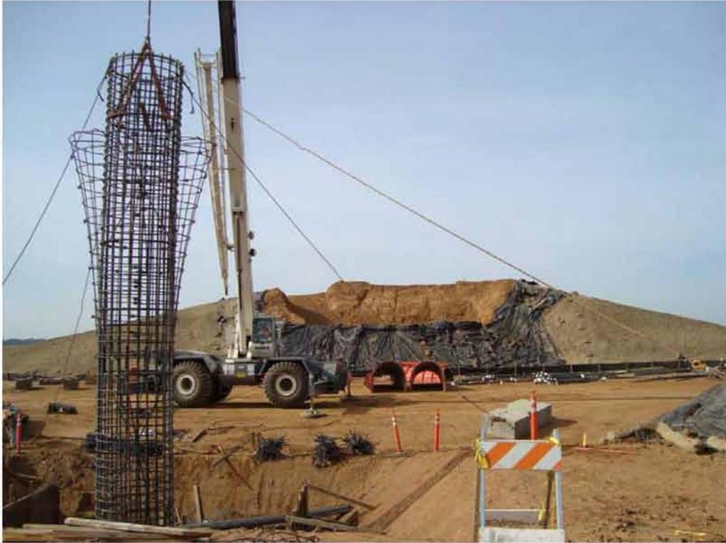
**Figure 1.10: Bridge Column Rebar Cage being held by a Crane**
