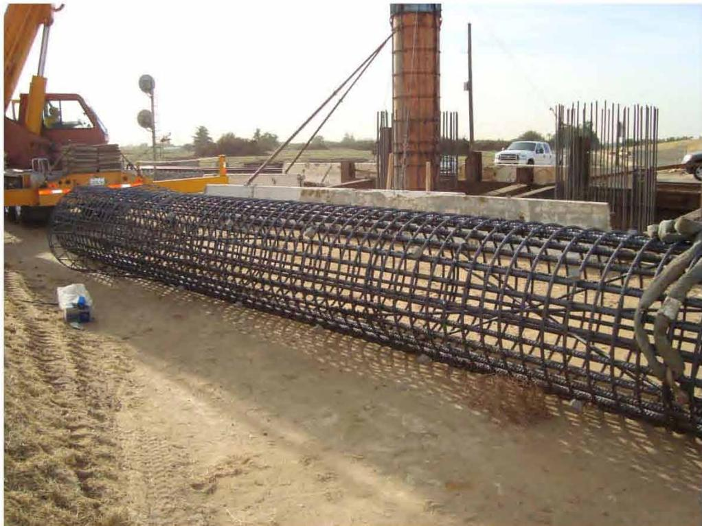
**Figure 2.17: Rebar Cage with two X-braces ready to be lifted**
