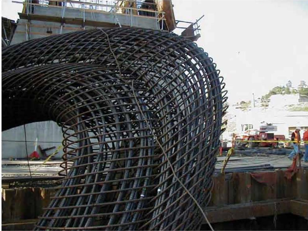
**Figure 1.5: No presence of Internal Braces in Bridge Column Rebar Cage in Bent 7 of Carquinez Bridge**
