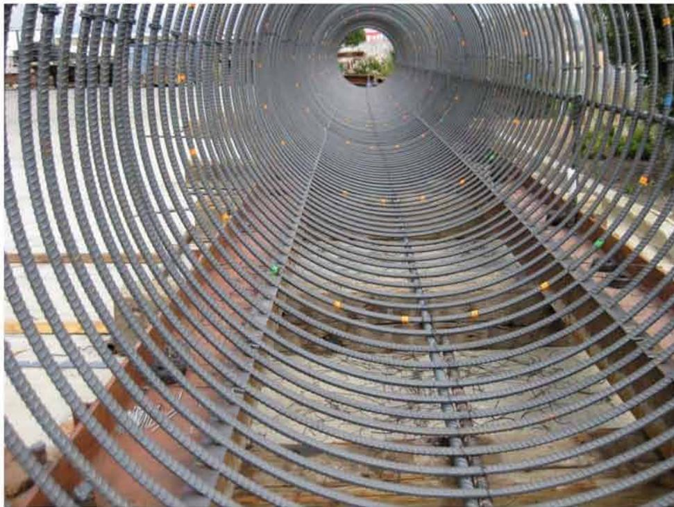
**Figure 2.1: Placing of Hoops for the Assembly of a Rebar Cage**
