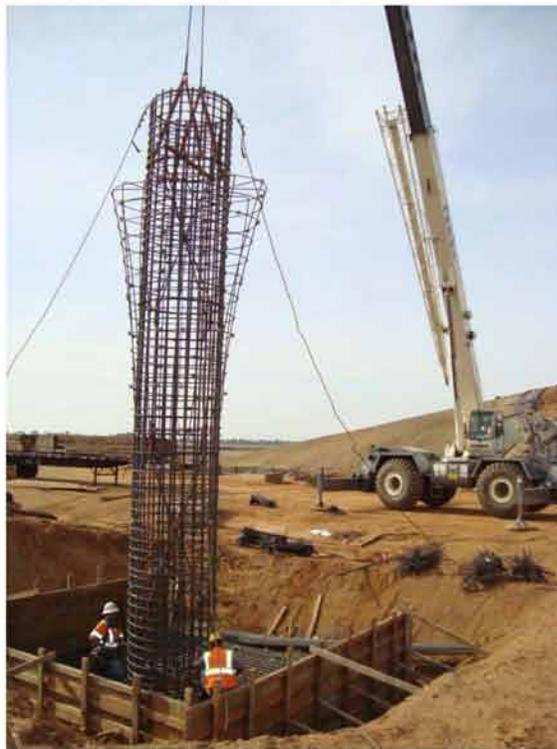
**Figure 2.23: Column Rebar Cage being Attached to the Bottom Mat of the Footing**
