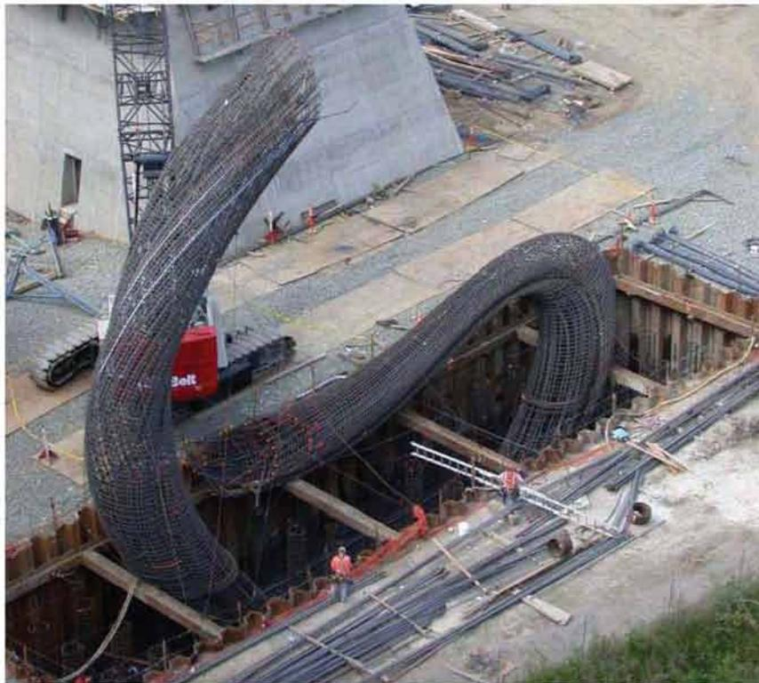
**Figure 1.2: Collapse of Bridge Column Rebar Cages in Bent 7 of Carquinez Bridge**
