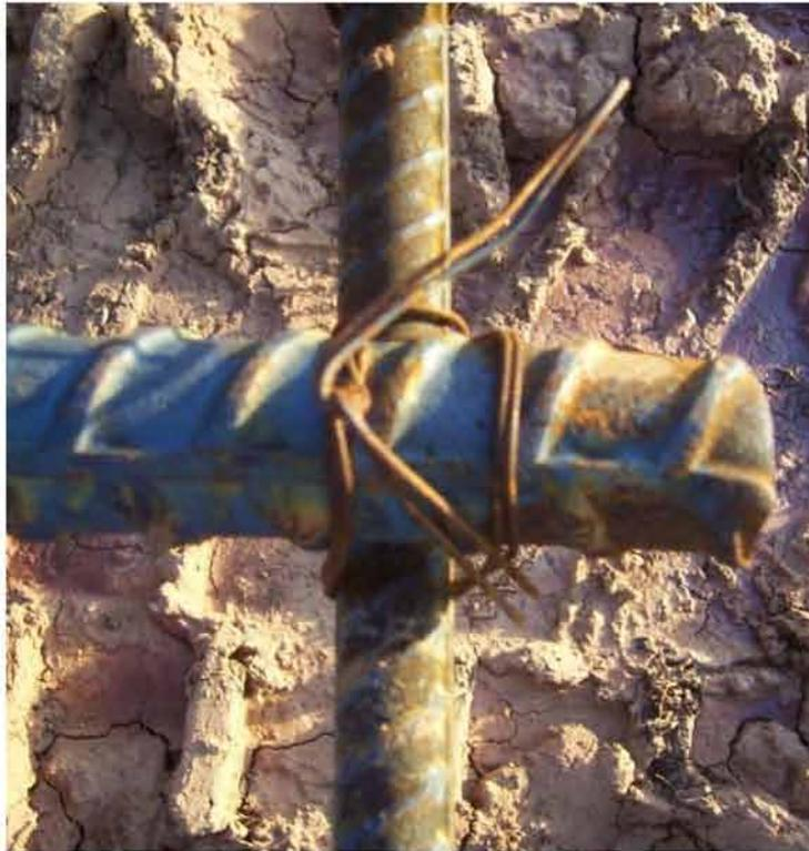
**Figure 2.9: Double-U Tie Wire Connection**
