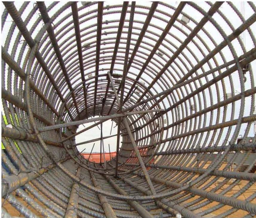
**Figure 2.15: Detail of Internal X-brace**
