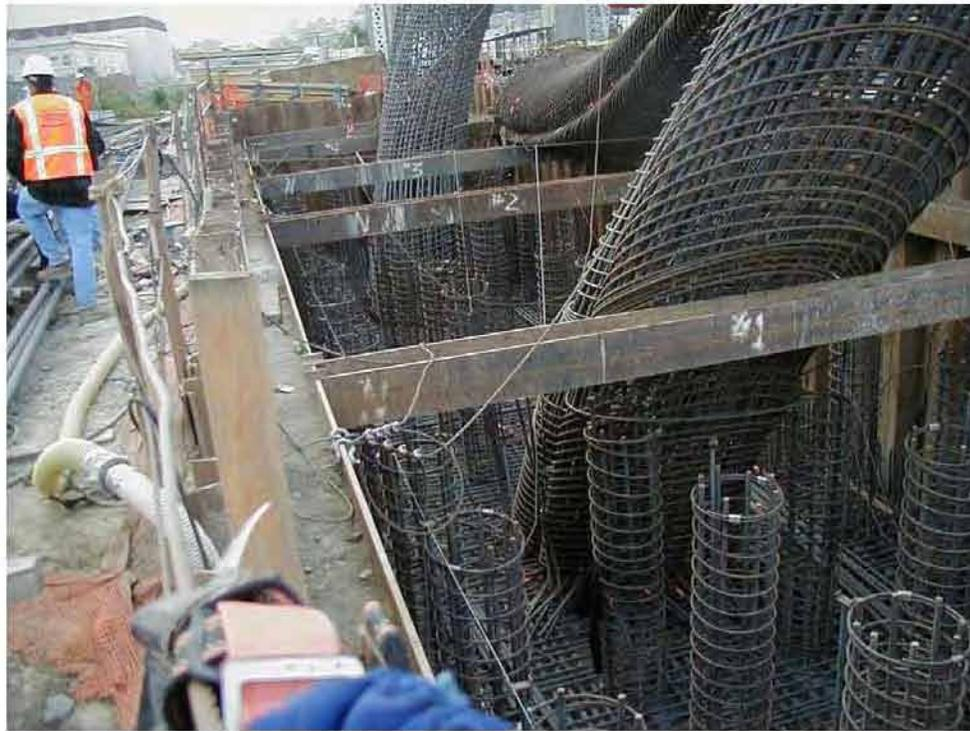
**Figure 1.3: Close-up of the footing for both Columns in Bent 7 of Carquinez Bridge**
