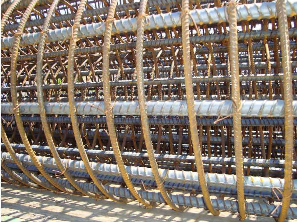
**Figure 2.14: Field-zone in a Column Rebar Cage**
