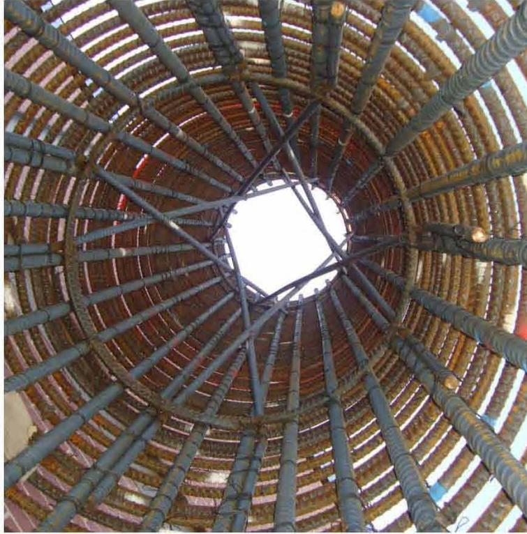
**Figure 2.16: Detail of Internal Square Brace**
