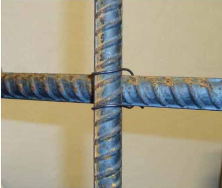
**Figure 2.8: Single-U Tie Wire Connection**
