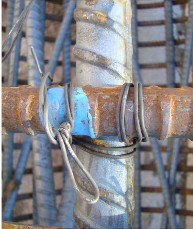
**Figure 2.10: Wrap-and-Saddle Tie Wire Connection**
