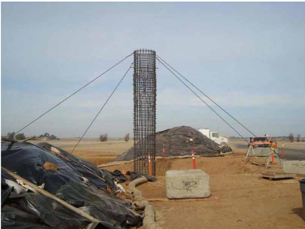
**Figure 2.27: Column Rebar Cage with four guy cables**
