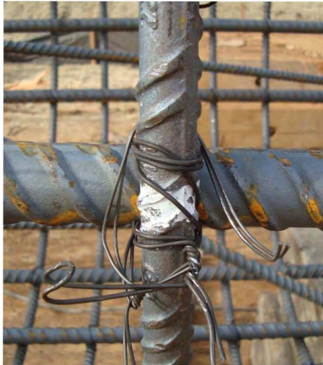
**Figure 2.12: Column-Tie Connection**
