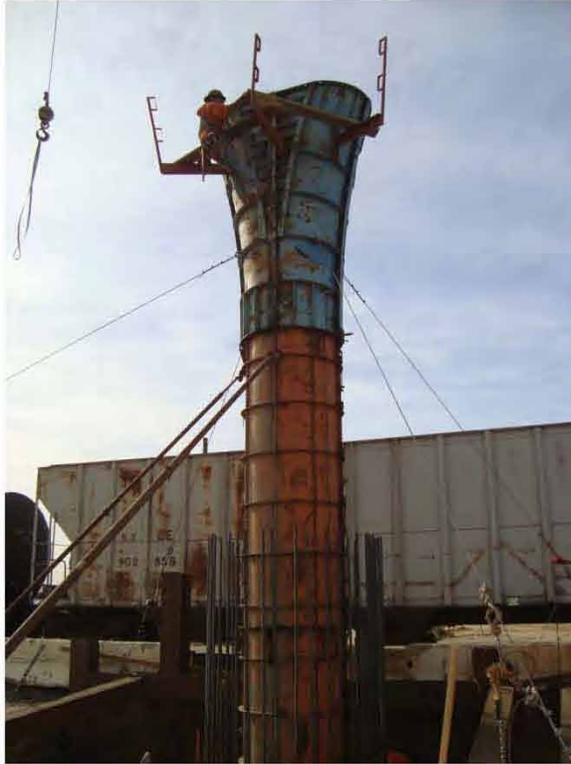
**Figure 2.18: Column Forms with Temporary Support installed**
