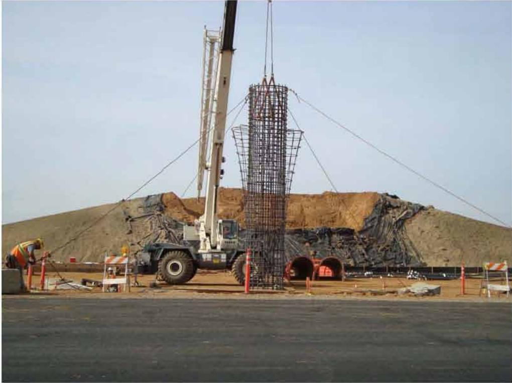
**Figure 2.24: Column Rebar Cage being guyed at four locations**
