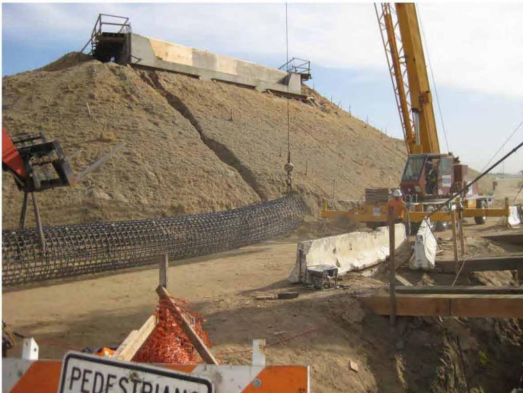
**Figure 2.19: Column Rebar Cage being lifted by the Crane with the help of a Forklift**
