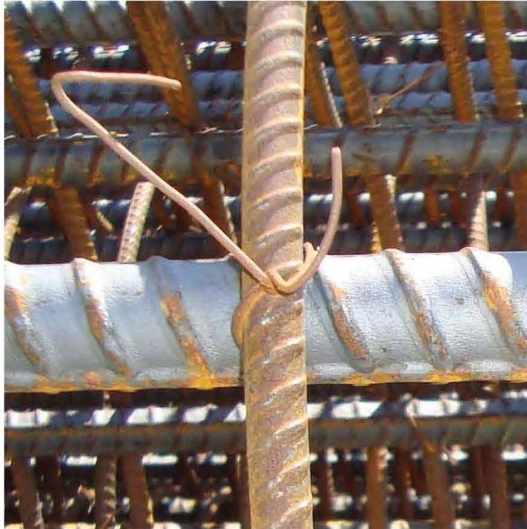
**Figure 2.6: Single-Snap Tie Wire Connection**
