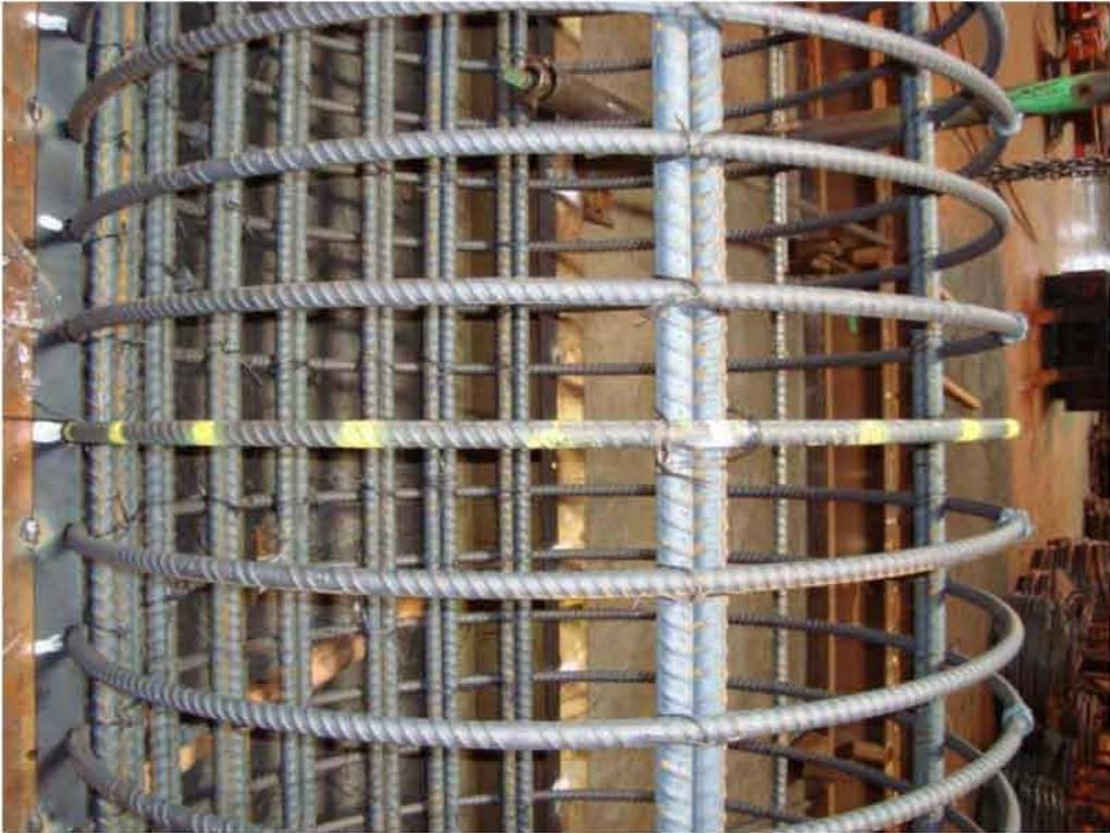
**Figure 2.3: Template-hoops in a Column Rebar Cage**
