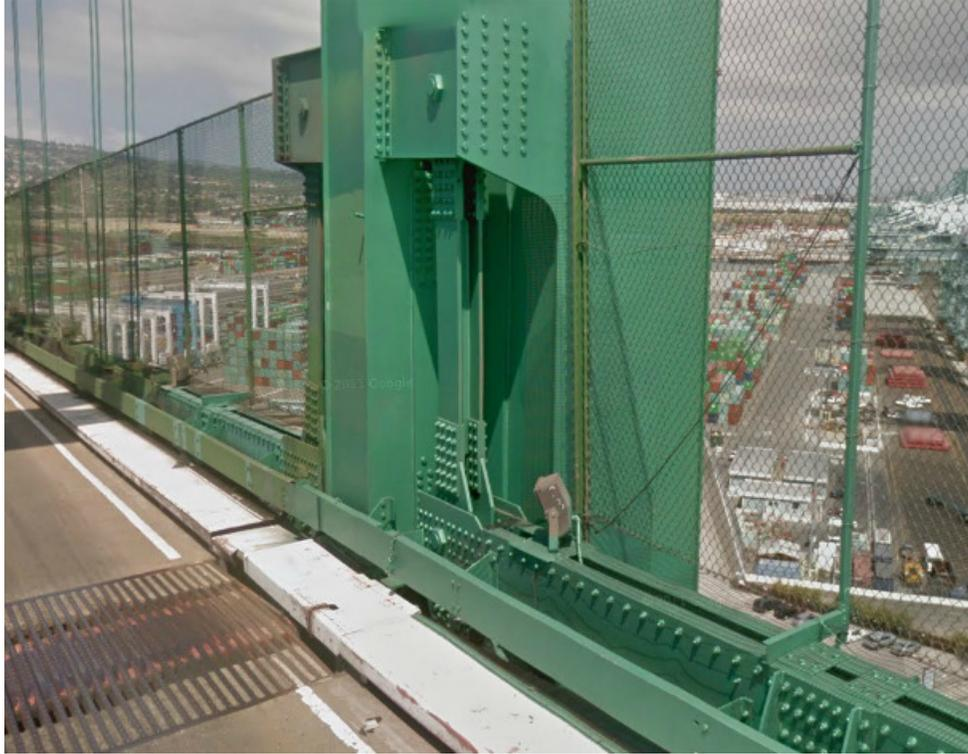
Figure C.10 Main and Side Span End Hinges
