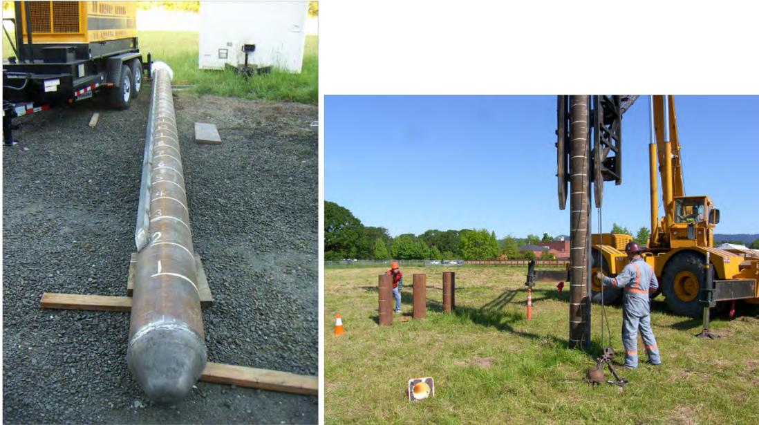
**Figure 4-11.** Installation of Baseline Pile (I-1)
