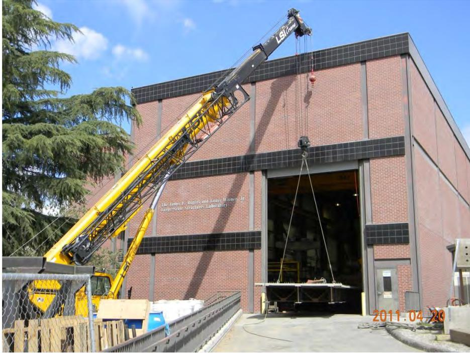
**Figure 4.5.11. Moving Superstructure Segment into the Laboratory**
