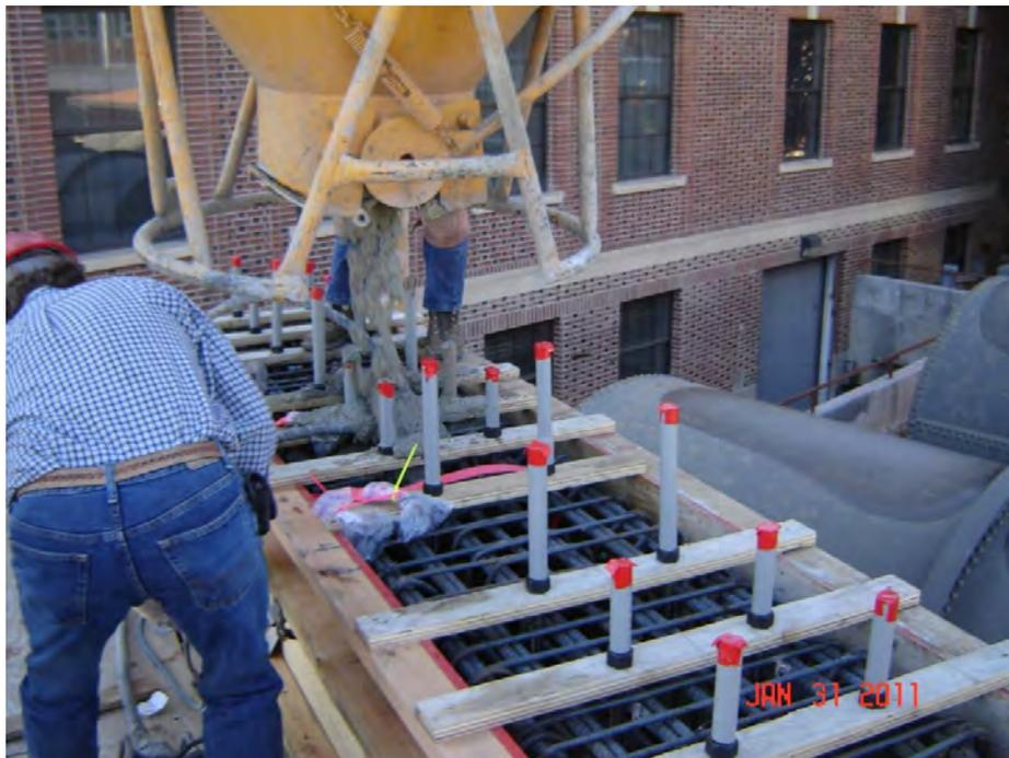
**Figure 4.5.6. Concrete Placement for Column and Bent Cap**
