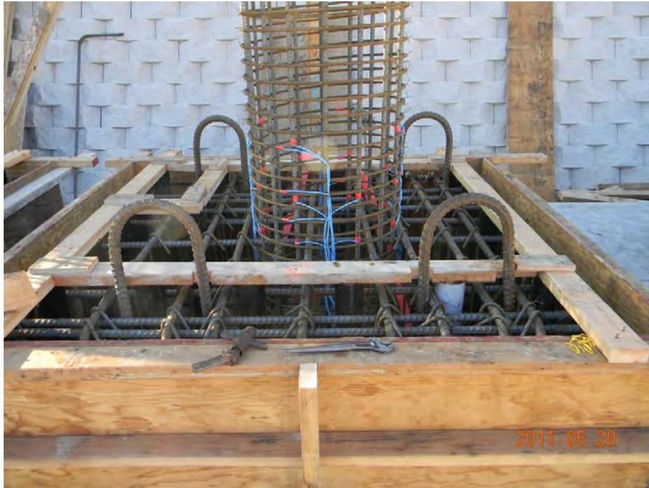
**Figure 4.5.3. Column Reinforcement Cage Placed in Footing Formwork**
