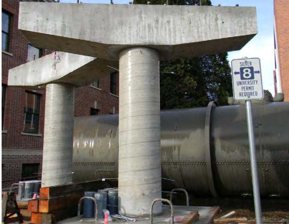
**Figure 4.5.7. Completed Single-Column Bents**
