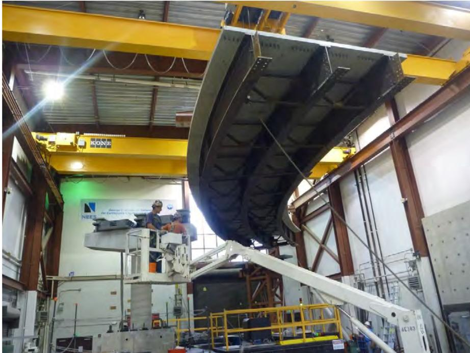
**Figure 4.5.12. Placement of North Segment of Superstructure**
