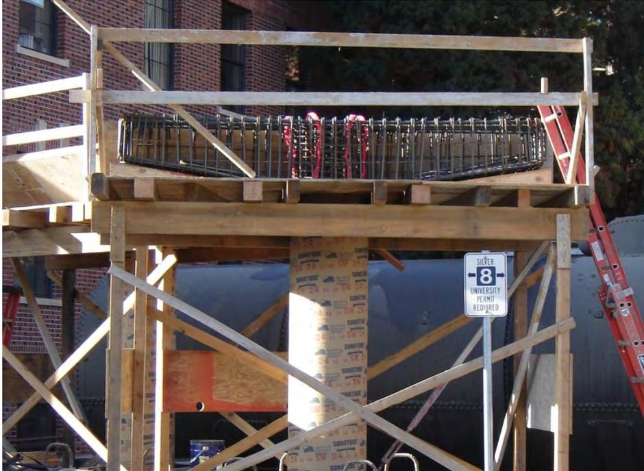
**Figure 4.5.5. Column Formwork and Bent Cap Reinforcement**
