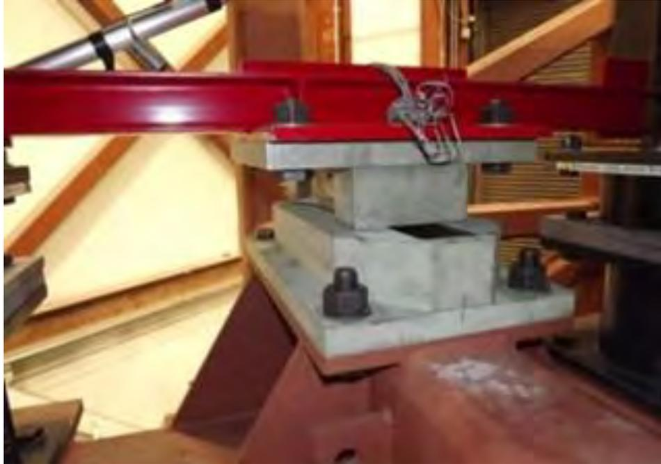
**Figure 4.4.4. Assembled Shear Key Installed Between Bottom Chord of Cross-Frame and Abutment Seat**
