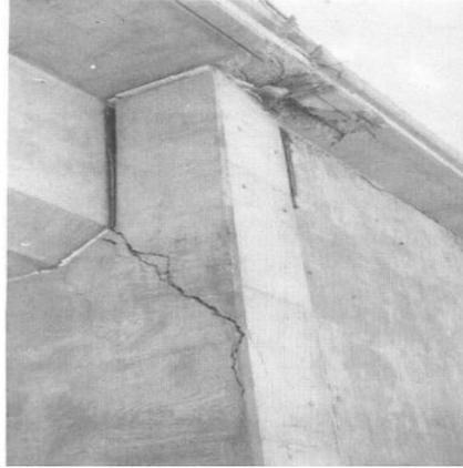
Figure 3-3. Damage state 5
