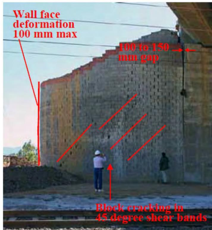
Figure 2.2. MSE wall at Muros Talca site showing deformations, permanent lateral displacement, and severe block cracking after 2010 Maule earthquake (Yen et al. 2011).
