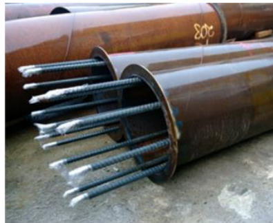
(b) welded dowels
