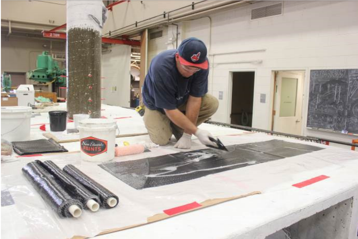
Figure 3.3 Coating the carbon sheets with epoxy resin and rolling the wet sheets in preparation for wrapping.
