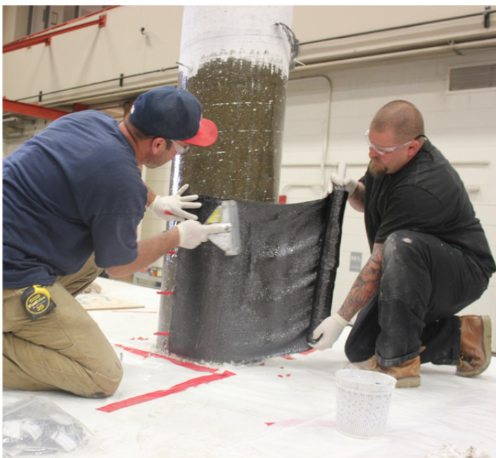
Figure 3.4 Applying the first CFRP layer of (a) the lower part of the jacket and (b) the upper part of the jacket of the column using the ready CFRP wet rolls.
