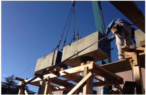
Fig. 2-25. Placing beam cap on the columns
