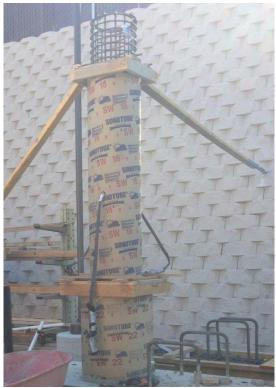
Fig. 2-23. Preparing the CIP columns
