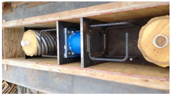
Fig. 2-24. Placing the load-cell, ducts and their spirals before placing the bar cage
