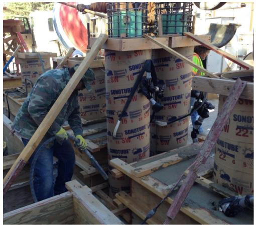
Fig. 2-20. Concrete cast for precast shells
