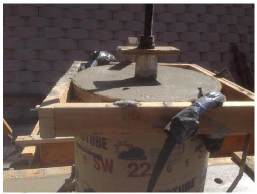
Fig. 2-21. Phase one concrete cast for BPSA
