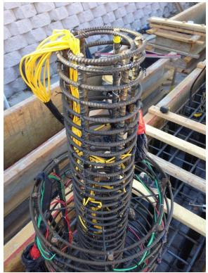
Fig. 2-49. Holding rebar-pin reinforcement cage stationary using welded rods
