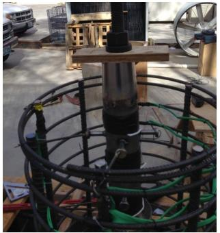
Fig. 2-19. Assembling the lower part of pipe-pin which embed in pedestal
