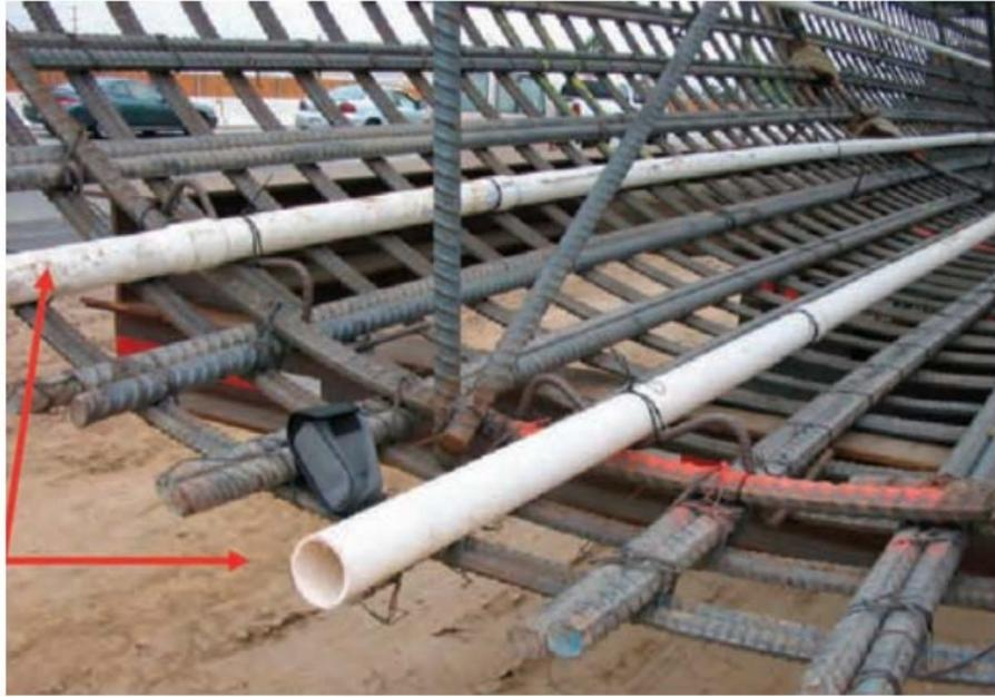
Figure 1.1 – Typical drilled shaft reinforcing cage with PVC inspection tubes (Alter 2011)
