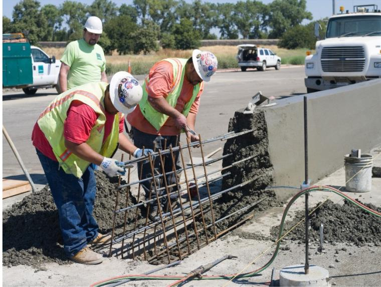
**Figure 2-6 Placing Rebar for the End Anchorage**
