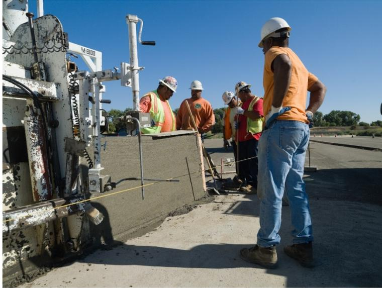
**Figure 2-4 Slip-forming the Barrier**
