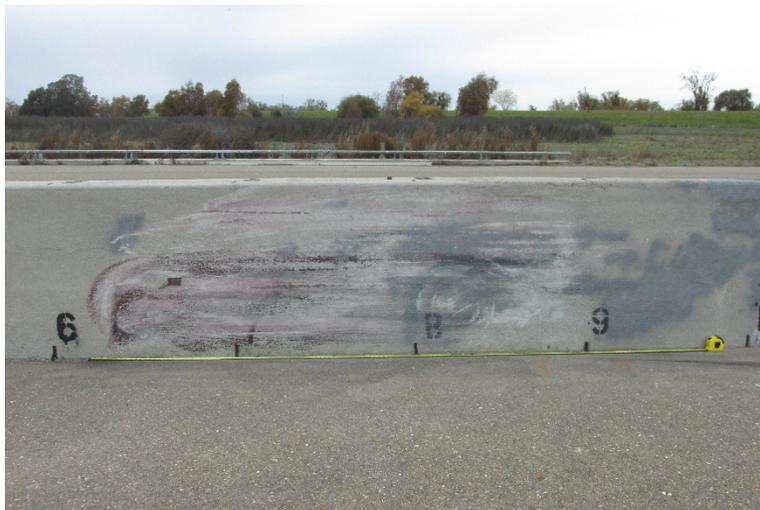
**Figure 5-6 Vehicle Marks on Type 60 Barrier**
