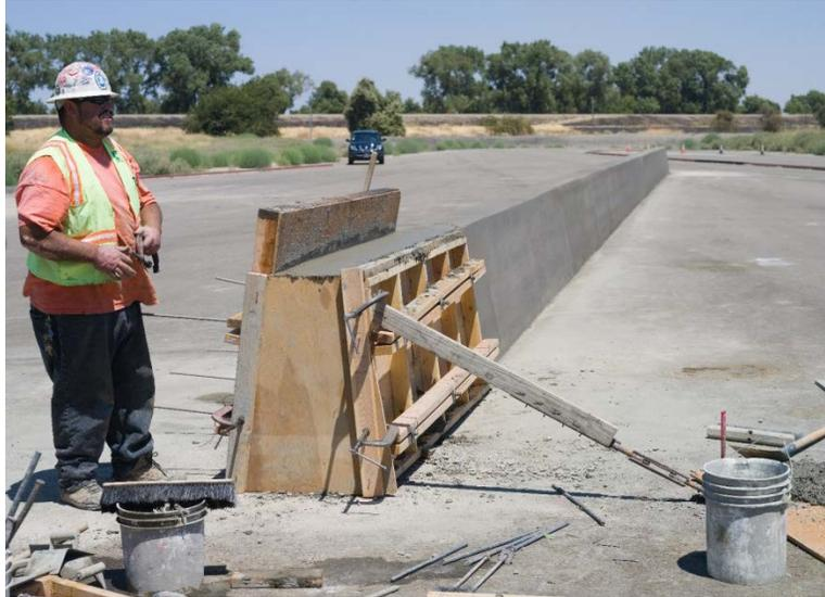
**Figure 2-8 End Anchorage Pour Complete**
