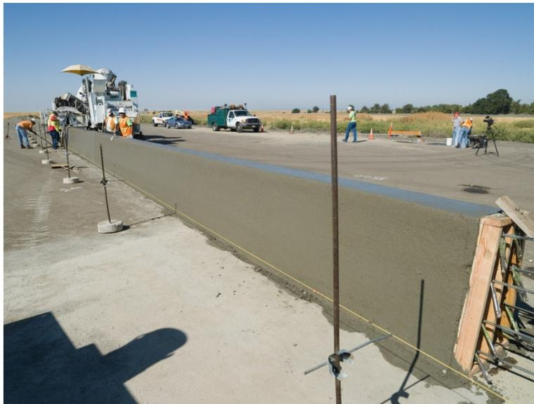
**Figure 2-5 Slip-forming Nearly Complete**
