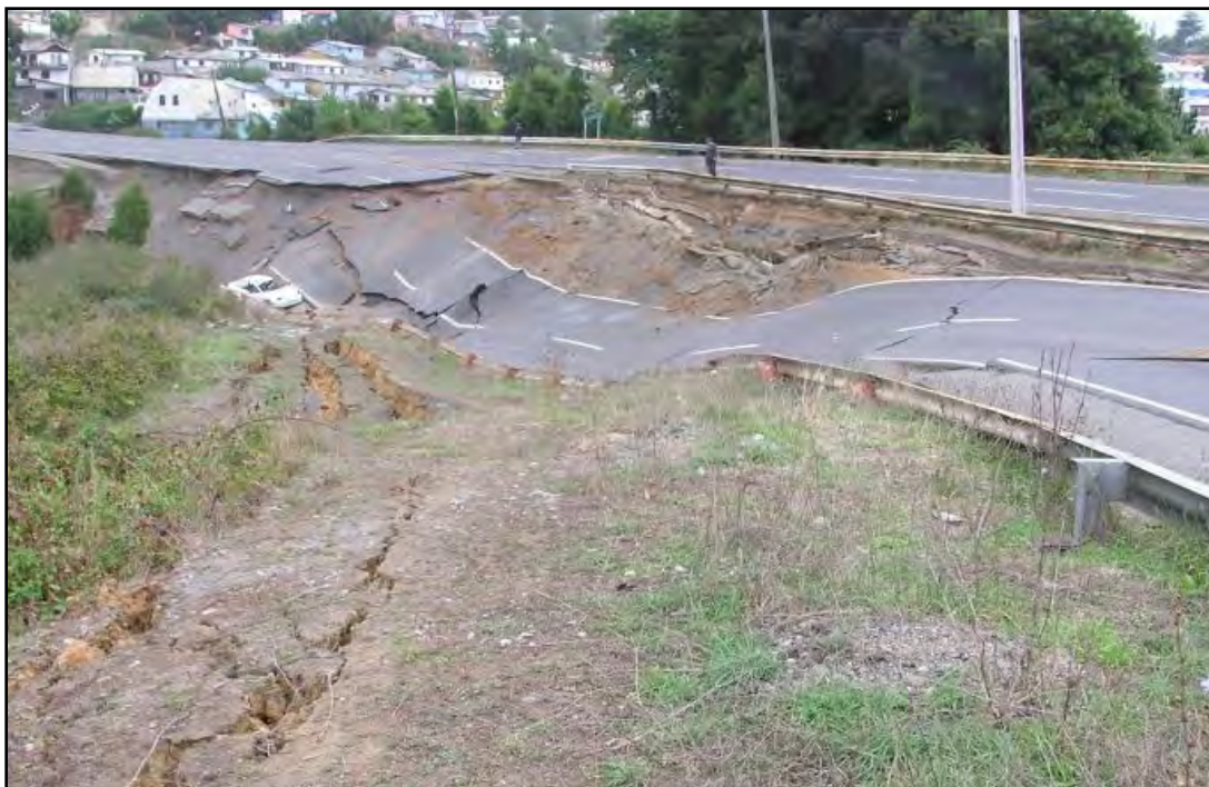
Slope failure on Route 160 in Lota, Chile following the M8.8 2010 Maule, Chile earthquake.
