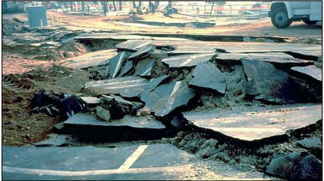
Ground failures in the 1994 Northridge Earthquake.
