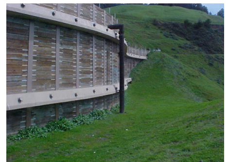
Timber lagging in a completed nongravity anchored wall.
