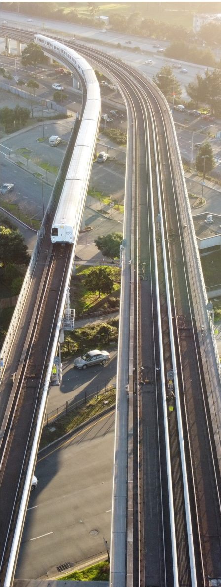
San Francisco Bay Area Rapid Transit (BART) train approaches Daly City Station.
