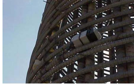
Figure 3.3.19 Installation of Signal Box for Conventional Strain Gauges
