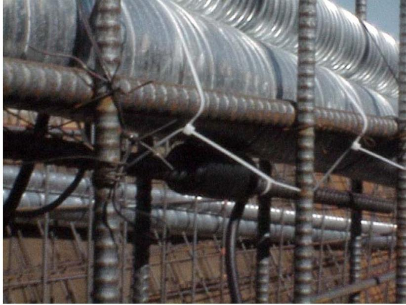
(a) LVDT Type Strain Meter Installed in the Deck
