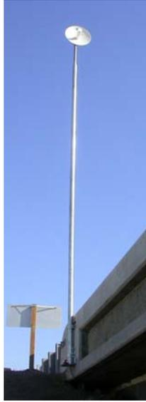
(a) Antenna mounted on a steel pole at JRO
