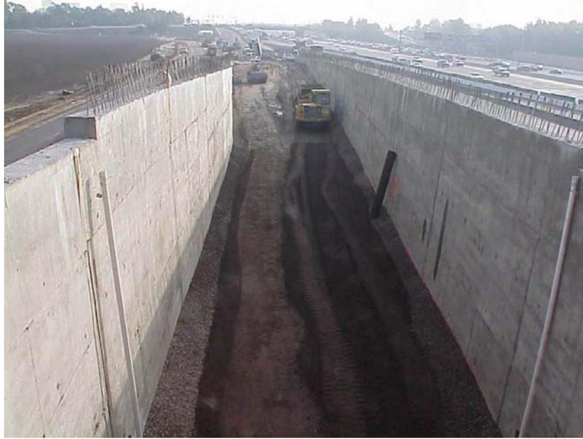
Figure 3.3.21 Backfilling at Abutment 1
