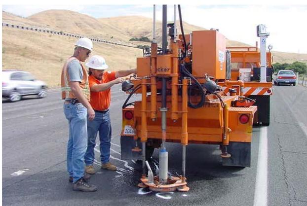
**Figure 6a. Coring Operation**
