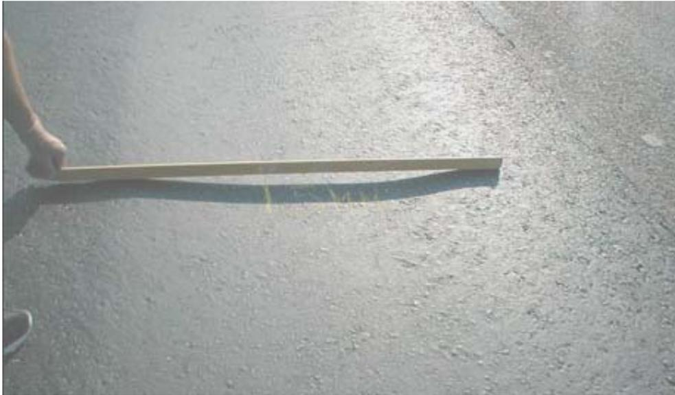
**Figure 5. Pavement Surface Rutting (over  $\frac{3}{4}$  inch) Suitable for Pulverization.**
