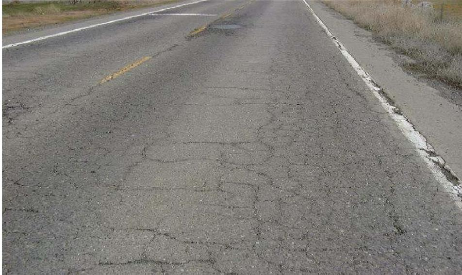
**Figure 4. Structurally Inadequate Pavement (severe alligator cracking and rutting distress) Suitable for Pulverization.**
