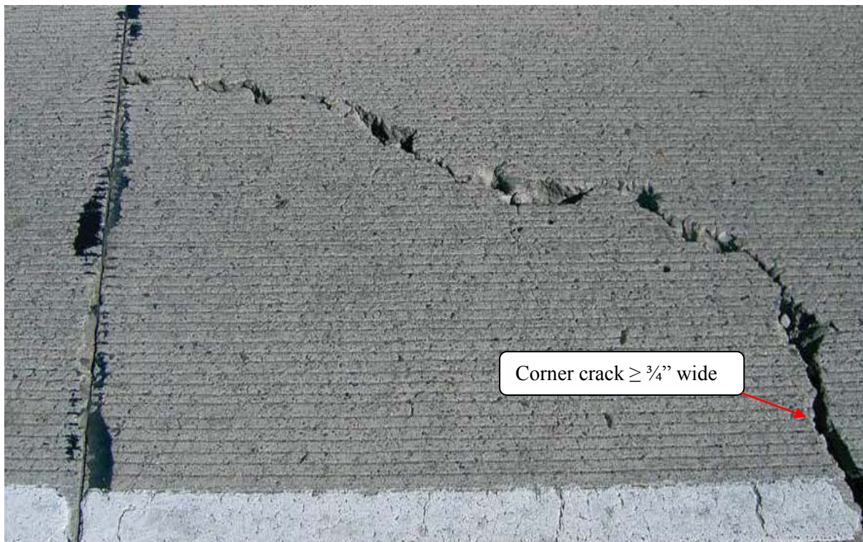
Figure 320-2: Replace slab – severe corner crack ≥ ¾" wide
