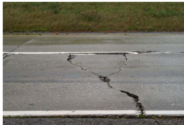
Figure 320-5: Replace slab and base – 3 rd stage cracking \geq \frac{3}{4} " wide, settlement \geq \frac{1}{4} ", spalling
