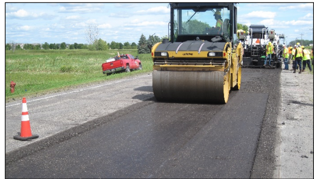
Figure 6.84: Primary compaction starting with smooth-drum roller on a PDR project.
