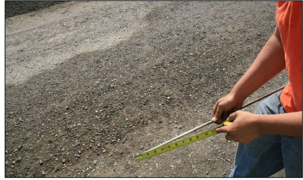
Figure 6.30: Measuring recycling depth on the T-bar (FDR).
