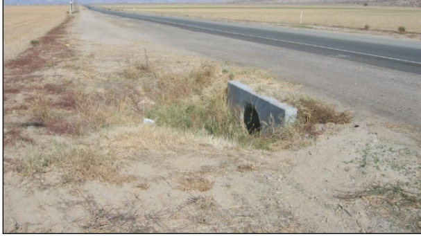
Figure 2.33: Blocked side drain and culvert.
