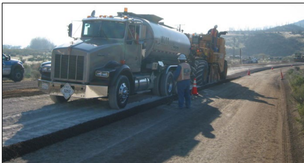
Figure 6.75: FDR-FA recycling train with no water tanker.
