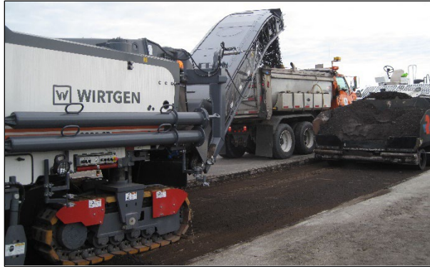
Figure 6.81: Removing excess material on a PDR project.
