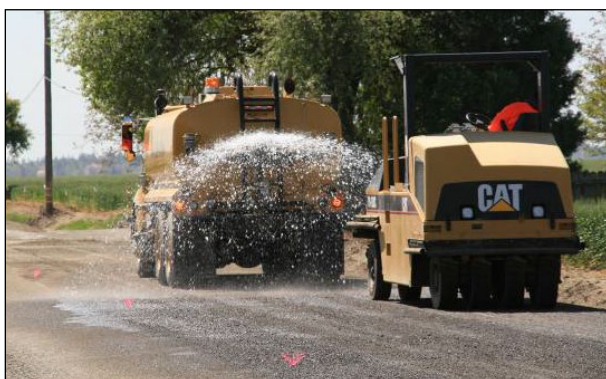
Figure 6.106: Final rolling on FDR projects with pneumatic-tired rollers.
