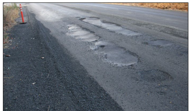
Figure 6.52: Trafficked recycled layer with severe raveling (patched) (PDR).
