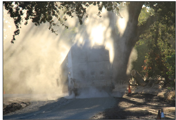
Figure 6.74: Loss of active filler/stabilizer during windy conditions.
