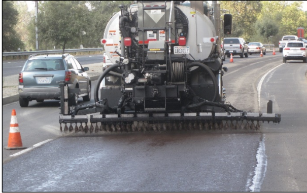
Figure 6.108: Curing seal application on a PDR project.
