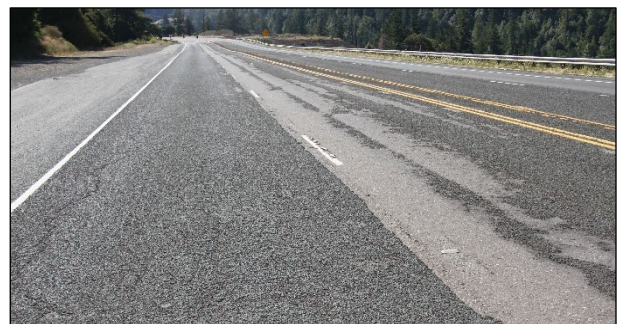
Figure 2.16: Example top-down distresses: Raveling.
