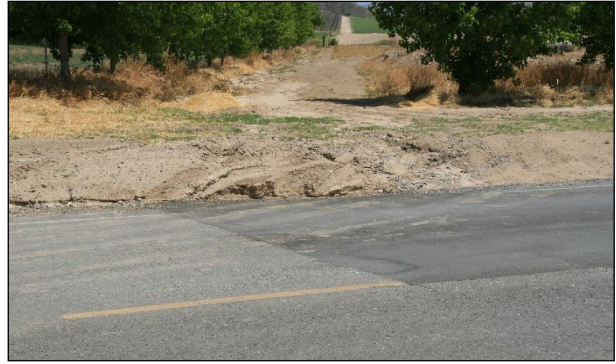
Figure 2.36: Access road drainage problems (note patch).
