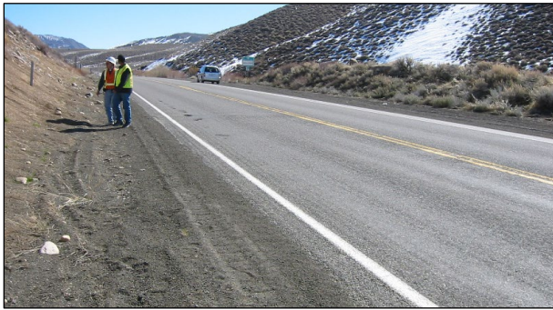
Figure 2.37: Absence of drains below cut slopes.
