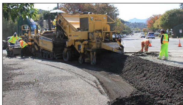
Figure 6.80: PDR project with pickup machine feeding the paver.
