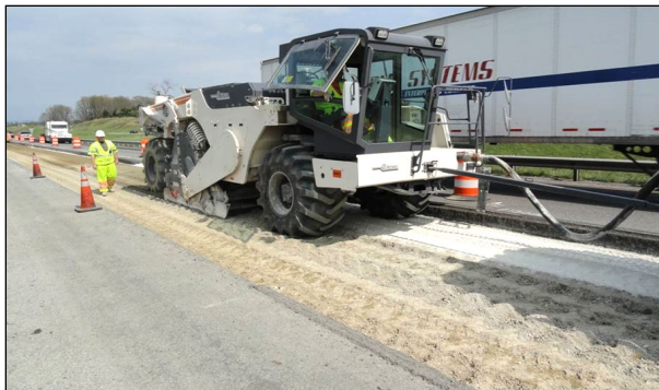
Figure 3.4: Stabilizing lower layers/subgrade prior to placing a CCPR layer.
