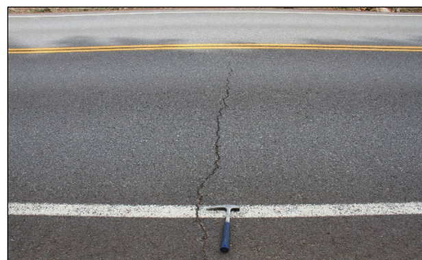
Figure 6.70: Reflected shrinkage crack in area of cement accumulation on an FDR-C project.
