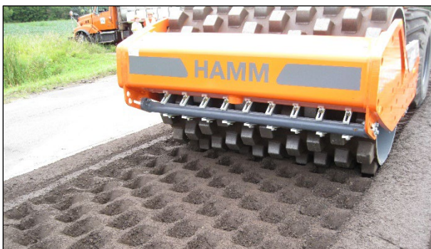
Figure 6.93: Padfoot impressions after first roller passes (FDR).
