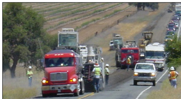
Figure 6.1: Pilot car traffic control on FDR project.
