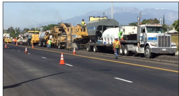
Figure 6.7: Multi-unit PDR recycling train.
