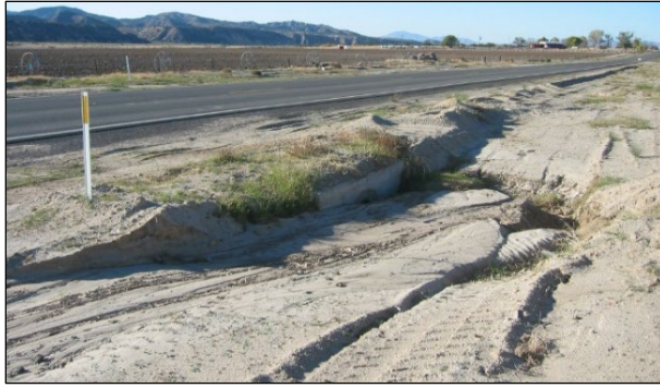
Figure 2.6: Example blocked side drains and culvert.
