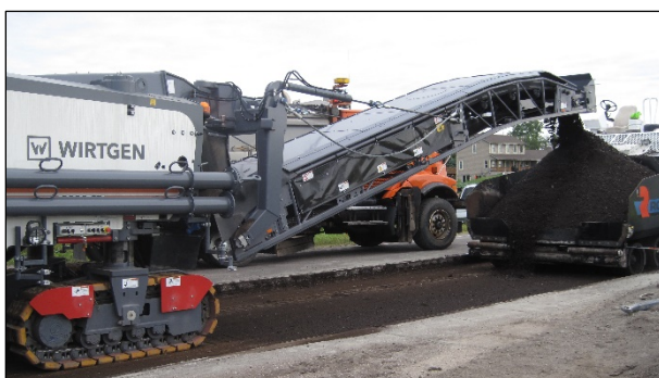
Figure 6.79: PDR project with belt feed into paver.
