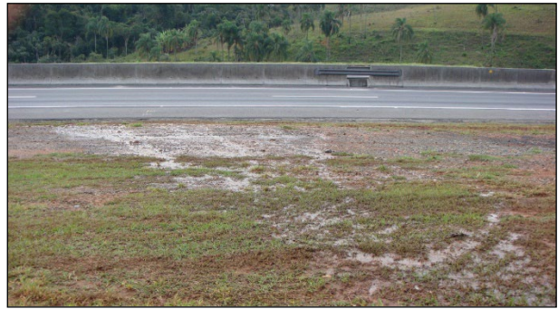
Figure 2.38: Water flowing downslope into the road.
