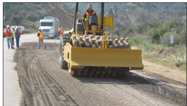
Figure 6.94: Padfoot impressions after multiple roller passes (FDR).
