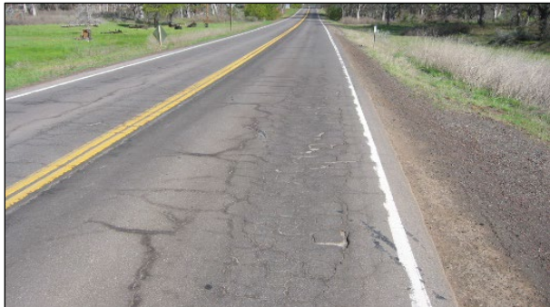
Figure 2.19: Example bottom-up distresses: Fatigue (alligator-B) cracks.
