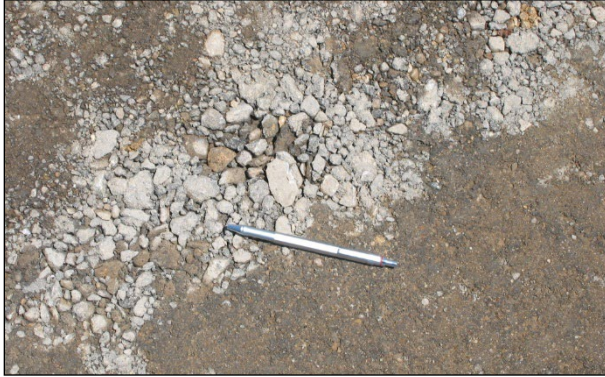
Figure 6.101: Segregation after excessive movement of material with a grader (FDR).
