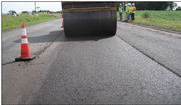
Figure 6.84: Primary compaction starting with smooth-drum roller on a PDR project.
