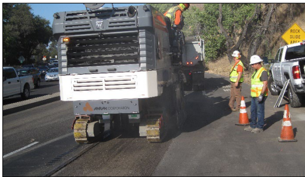
Figure 6.2: Premilling to maintain crossfall prior to PDR.
