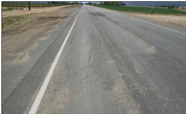
Figure 2.31: Early failure in wheelpath repairs.
