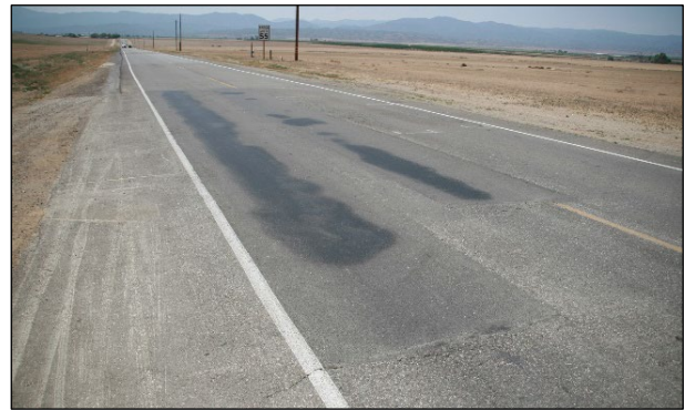
Figure 2.32: Bleeding in wheelpath repairs.
