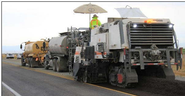
Figure 1.2: Partial-depth recycling train (single unit).
