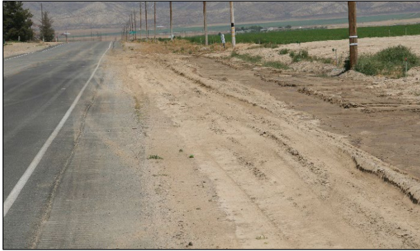
Figure 2.35: Irrigation water sprays on the road or unpaved shoulder.
