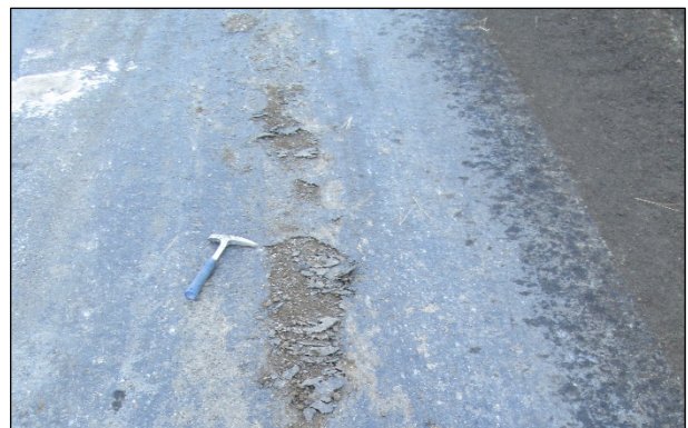
Figure 6.118: Delaminated area exposed during shrinkage crack mitigation (FDR-C).
