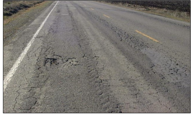
Figure 2.30: Fatigue cracking and potholes in wheelpath repairs.
