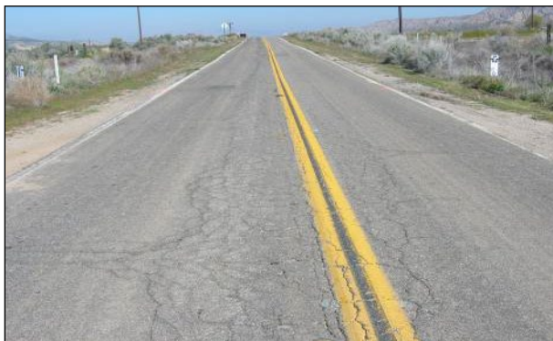
Figure 2.4: Example alligator-B cracking.
