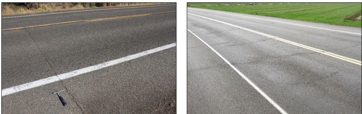
Figure 3.7: Reflected shrinkage cracks on FDR-C projects.
