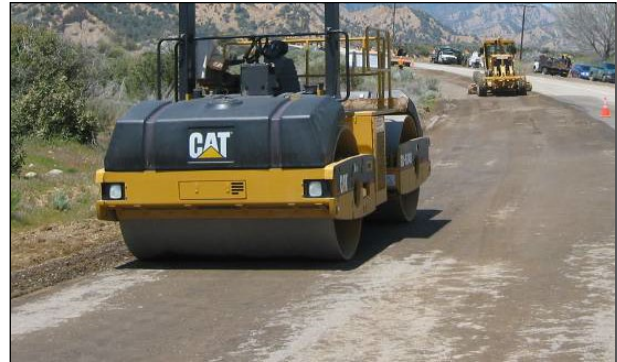
Figure 6.104: Intermediate rolling on FDR layer with double drum steel roller.
