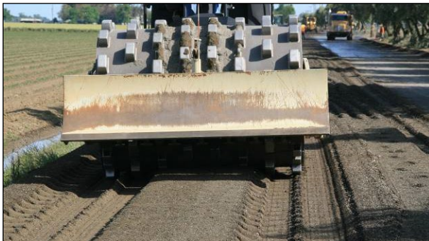
Figure 6.91: First padfoot roller pass on an FDR project.
