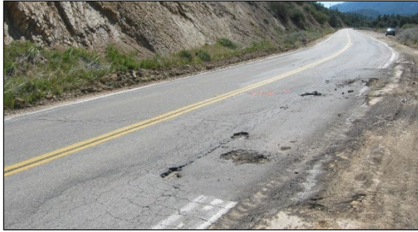
Figure 2.17: Example top-down distresses: Potholes.
