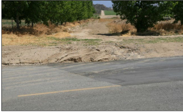
Figure 2.2: Example road below natural ground level.
