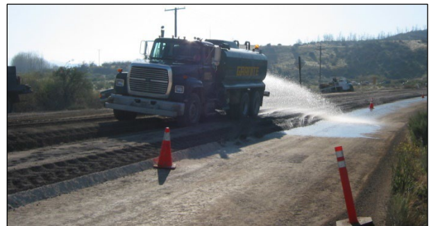
Figure 6.76: Separate water application behind recycler (FDR).
