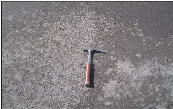
Figure 6.49: Good quality PDR and FDR surfaces after final compaction.
