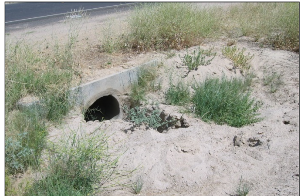
Figure 6.124: Soil blocking a culvert after completing an FDR project.
