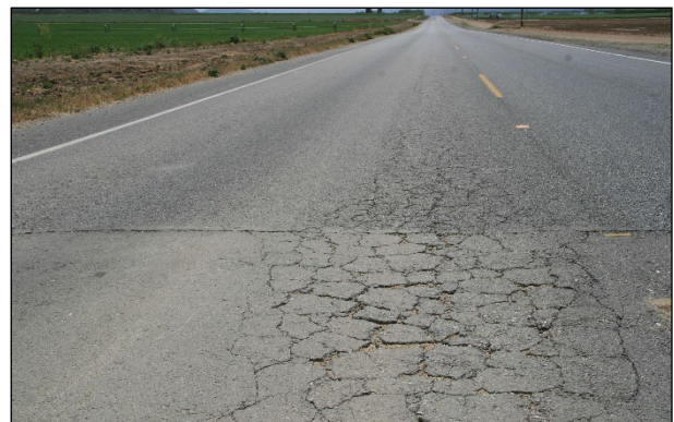
Figure 2.28: Early failure in patch (drainage problem).
