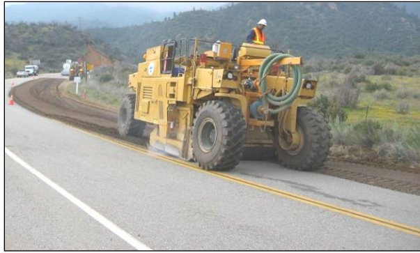
Figure 6.55: Prepulverization on an FDR project.
