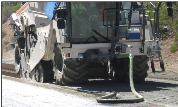
Figure 6.21: Water leak during tanker change (FDR).
