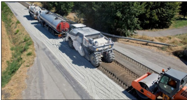
Figure 6.8: Wheel-driven FDR recycling train.
