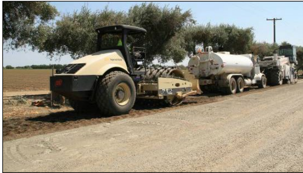
Figure 6.95: Primary compactor working in close proximity to recycling train (FDR).
