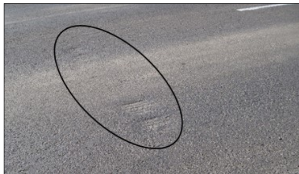
Figure 6.112: Permanent truck tire impressions on a PDR layer.
