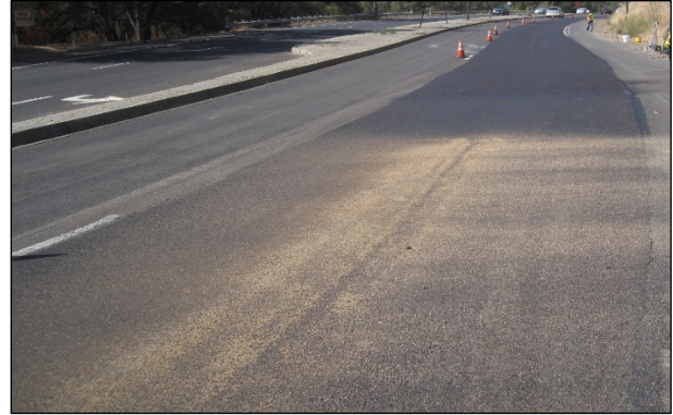
Figure 6.109: Curing seal after application of sand on a PDR project.
