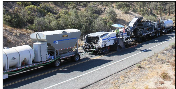
Figure 1.3: Partial-depth recycling train (multi-unit).
