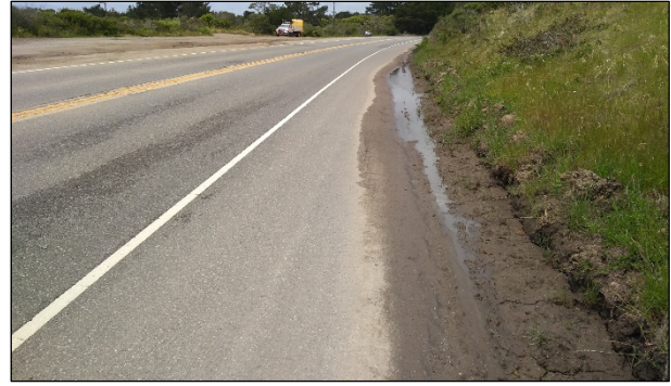
Figure 2.7: Example drainage problem in cut.
