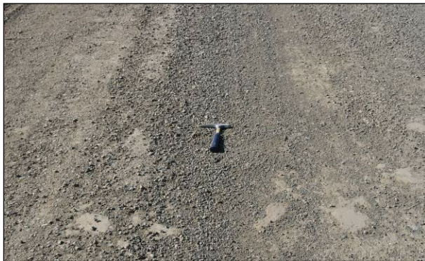
Figure 6.50: Unacceptable PDR and FDR surfaces after final compaction.
