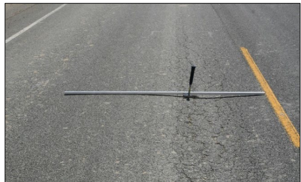
Figure 2.5: Example rutting associated with base/subgrade failure.
