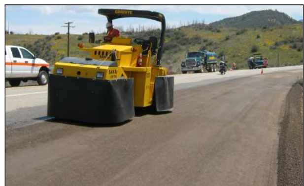
Figure 6.106: Final rolling on FDR projects with pneumatic-tired rollers.
