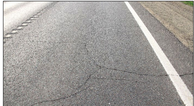
Figure 2.20: Example bottom-up distresses: Block cracks.
