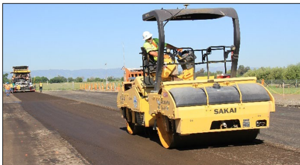
Figure 6.13: Steel breakdown roller on a PDR layer.
