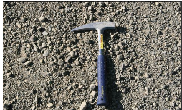
Figure 6.50: Unacceptable PDR and FDR surfaces after final compaction.
