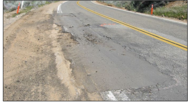
Figure 2.18: Example top-down distresses: Edgebreak.
