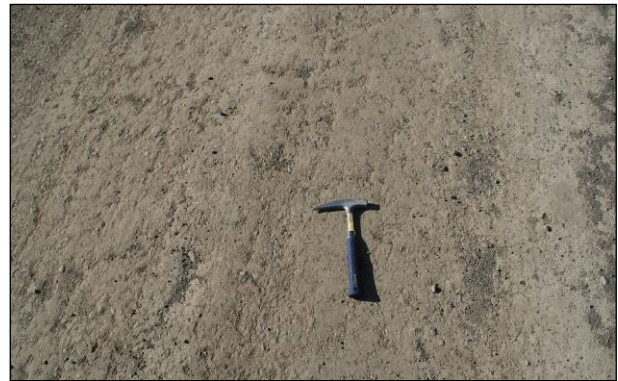
Figure 6.49: Good quality PDR and FDR surfaces after final compaction.
