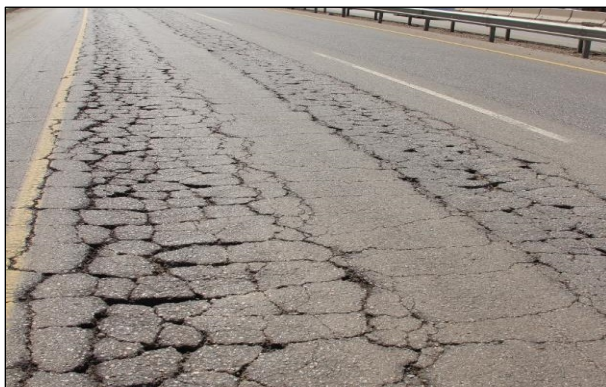
Figure 2.27: Loose blocks in severe alligator-B cracking.
