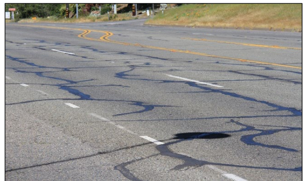
Figure 2.24: Example bottom-up distresses: Sealed reflective cracks.
