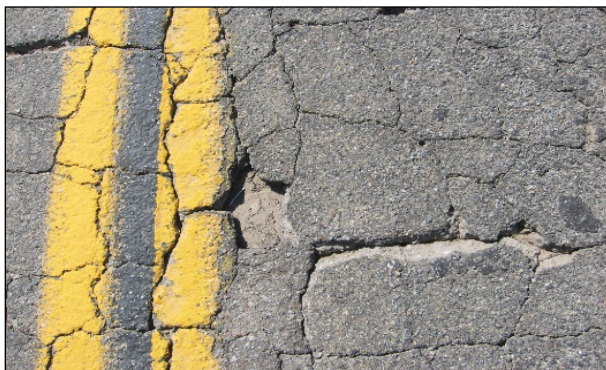
Figure 2.23: Example bottom-up distresses: Unsealed reflective cracks.
