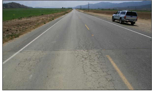
Figure 2.3: Example early full-width patch failure.
