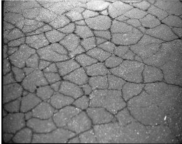
Localized High Severity Alligator Cracking
