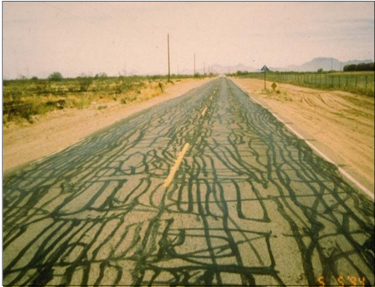
EXCESSIVE SEALANT
