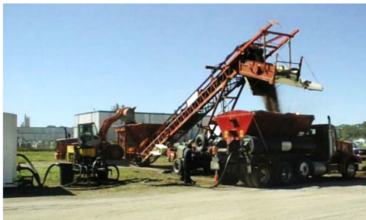
Figure 9-12 A Typical Project Staging Area (SlideServe)
