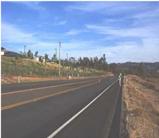
a) High Quality Longitudinal Joint
