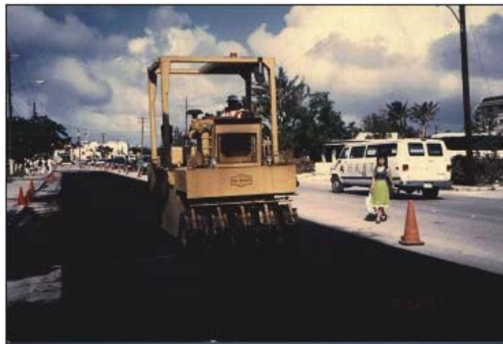
Figure 9-25 Rolling a Micro Surfacing
