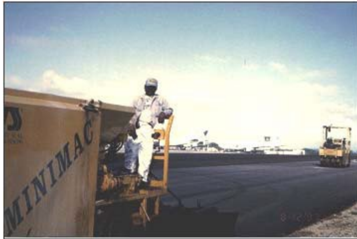
Figure 9-26 Rolling of Micro Surfacing on Airport Taxiways
