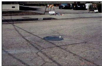
c) Cover Utilities with Kraft Paper
