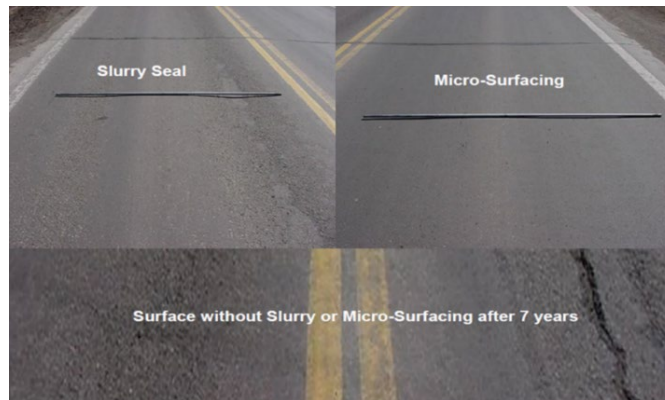
Figure 9-3 Comparison of Distresses after 7-Years in High Mountain Climate Region
