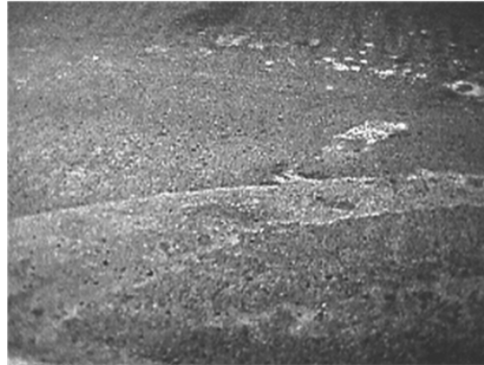
Figure 8-25 Damage Due to Post Application Heavy Rain with Shear
