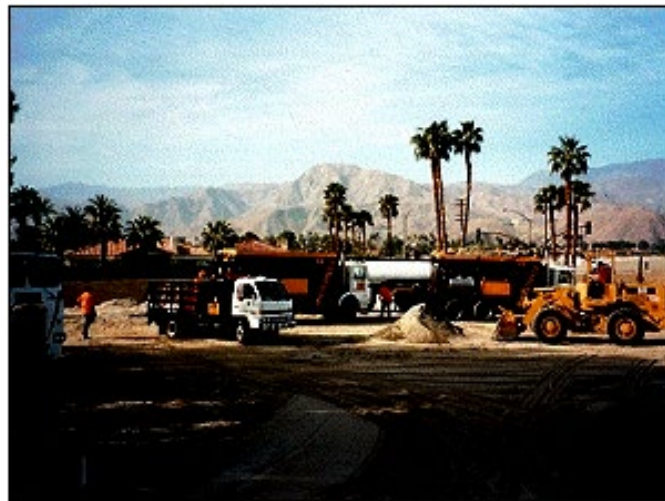
Figure 8-16 A Typical Stockpile and Project Staging Area
