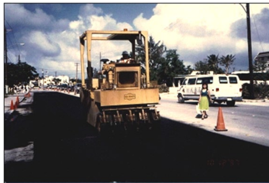
Figure 8-26 Rolling a Slurry Surfacing
