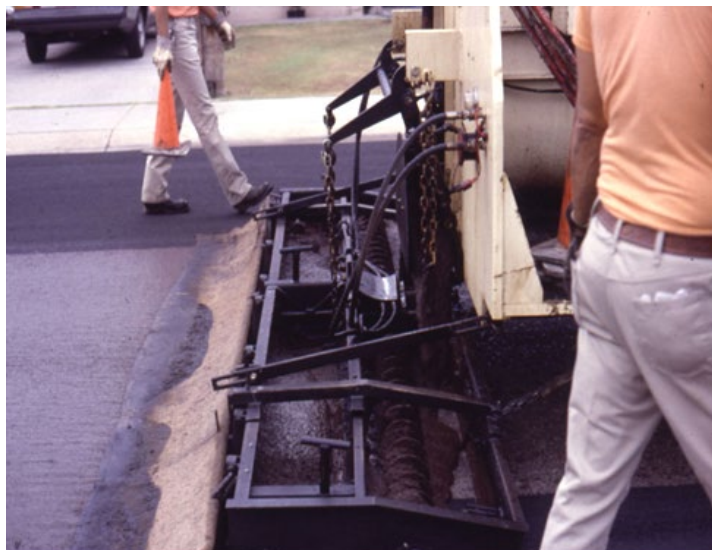
Figure 8-9 Slurry Seal of Micro Surfacing Box with Augers
