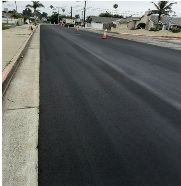
Figure 8-10 HB Hi-Mod Slurry Seal, CP2 Center, 2024 (Courtesy of Erik Updyke)
