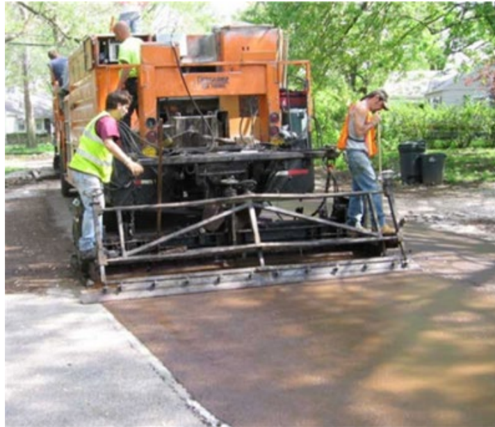
Figure 8-8 Slurry Surfacing Machine
