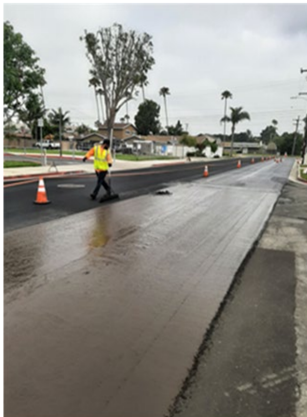
Figure 8-11 HB Hi-Mod Slurry Seal CP2 Center, 2024 (Courtesy of Erik Updyke)
