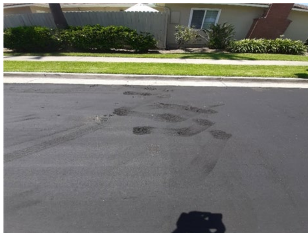
Figure 8-13 Example of Scuffing from Early Traffic on HB Hi-M
