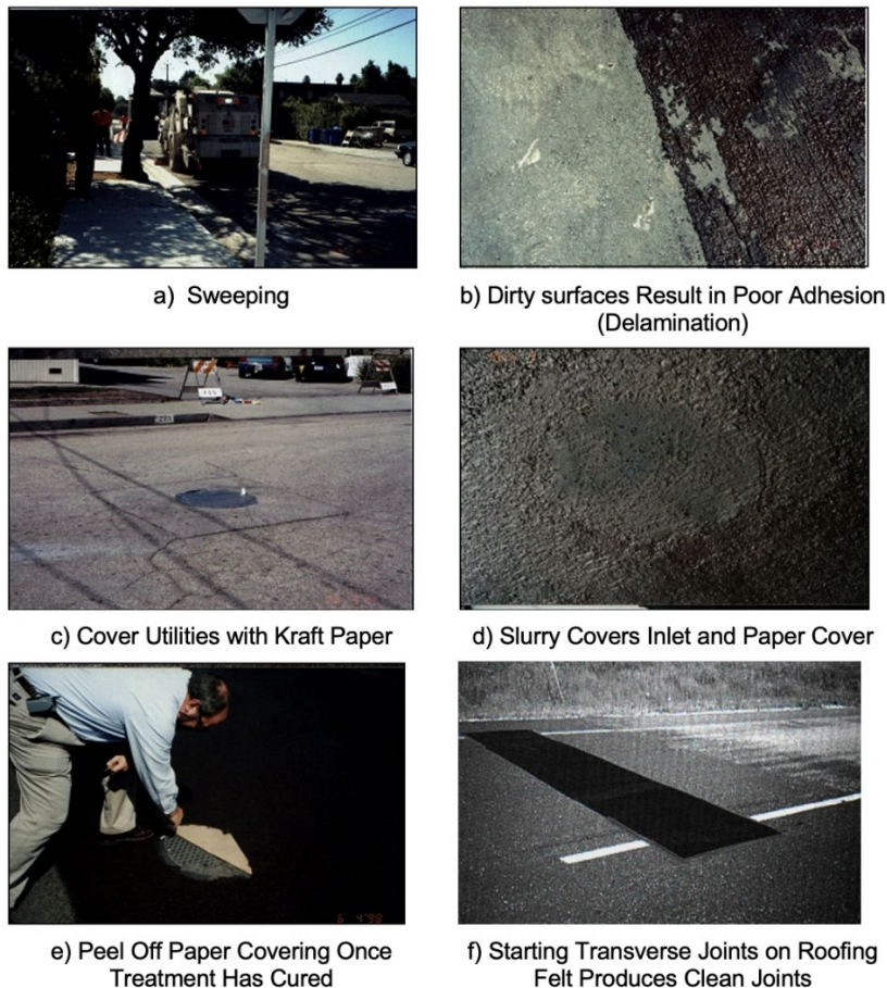
Figure 8-17 Surface Preparation Methods
